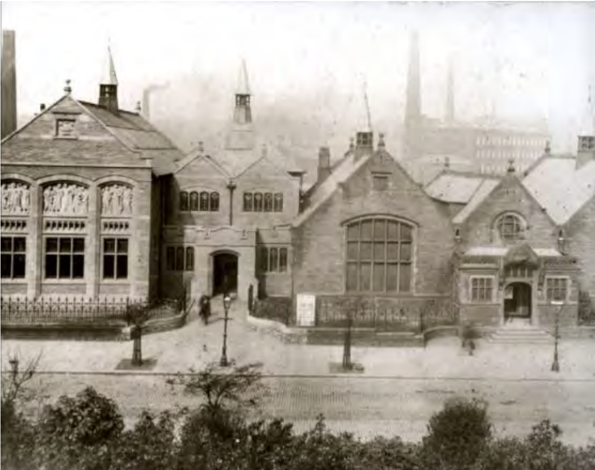
Fig.10 Above: Photograph Showing First & Second Phases
