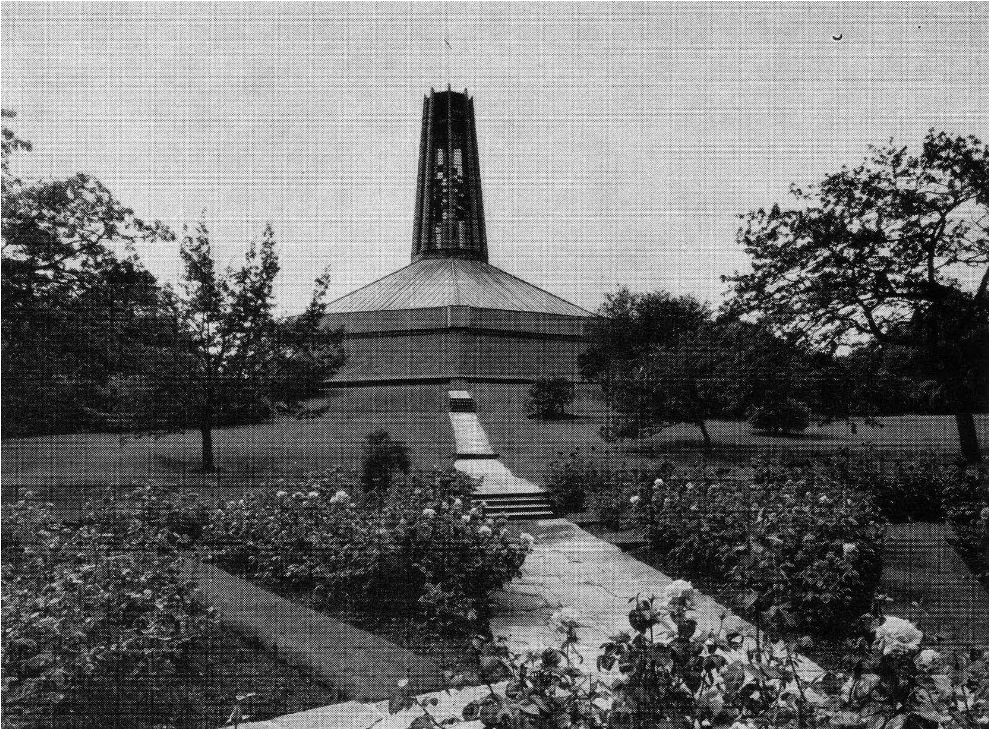
Figure 3.4 Chapel viewed from Hopwood Hall (Source: Rochdale Archives)
