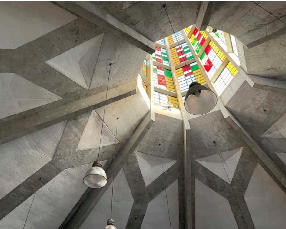
1 View looking up towards stain glass window.
