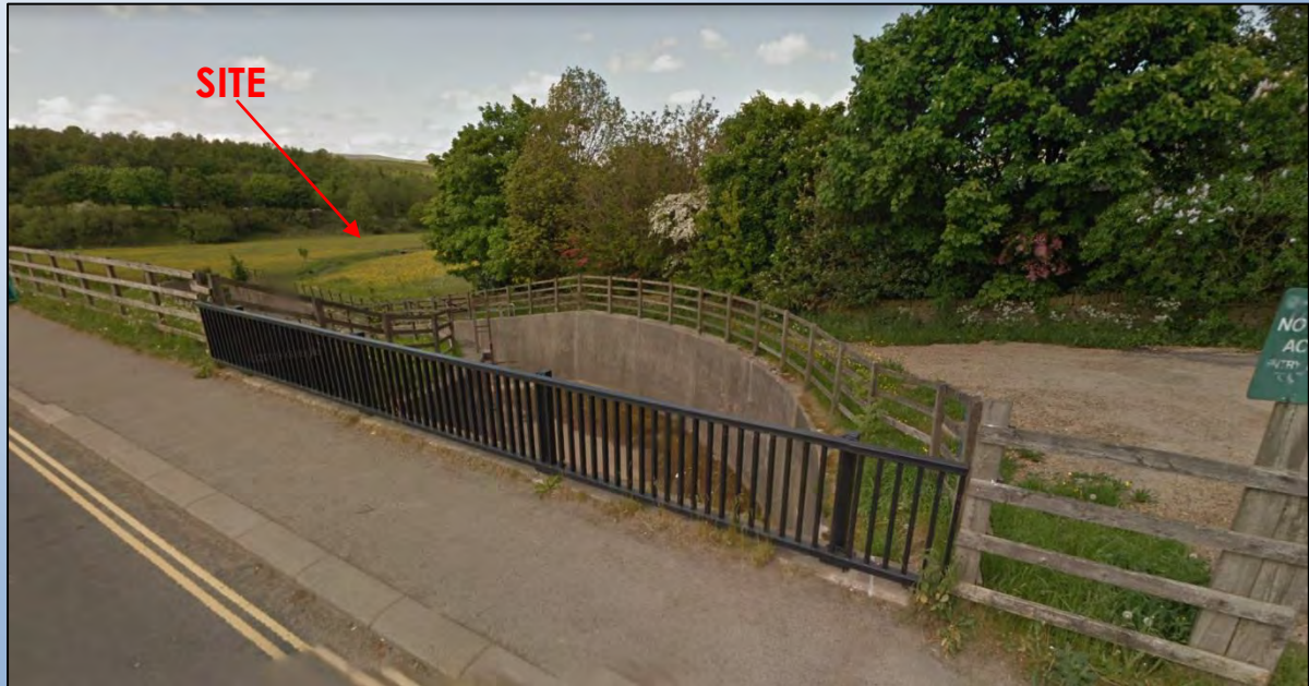
Figure 5: Concrete Overflow Channel – Hollingworth Brook (Google, 2023)
