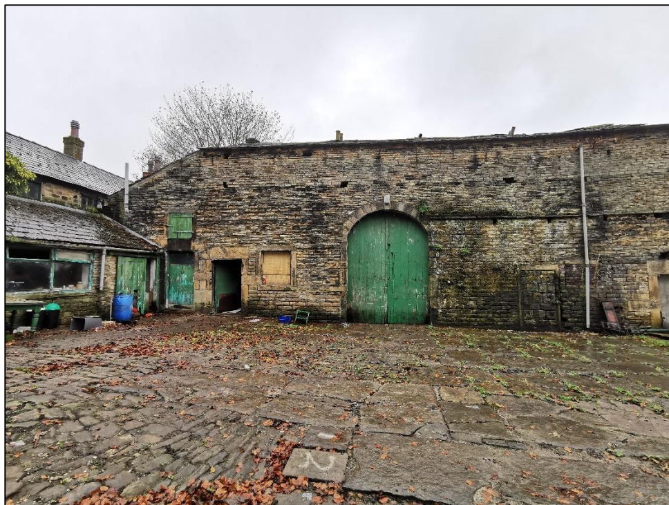
Plate 1 - Barn as viewed from the south looking north view 1
