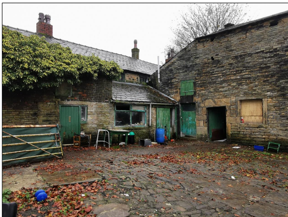
Plate 8 - Where the barn meets the dwelling (not surveyed) on the western aspect
