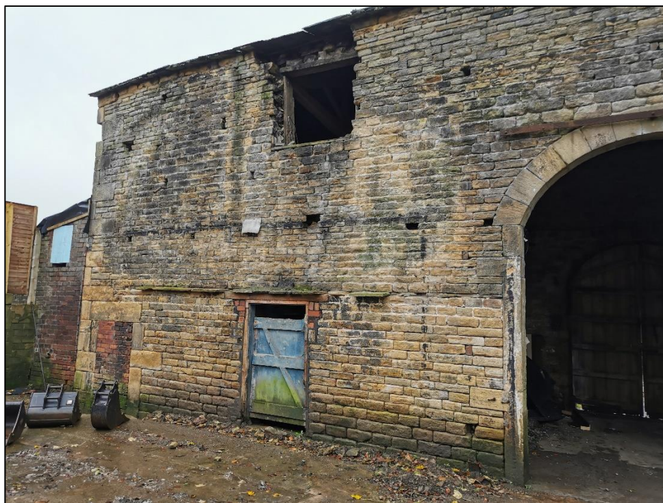
Plate 3 - Barn as viewed from the north looking south view 2
