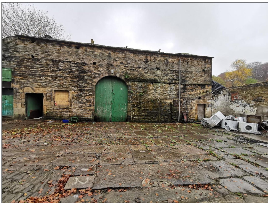
Plate 4 - Barn as viewed from the north looking south view 2
