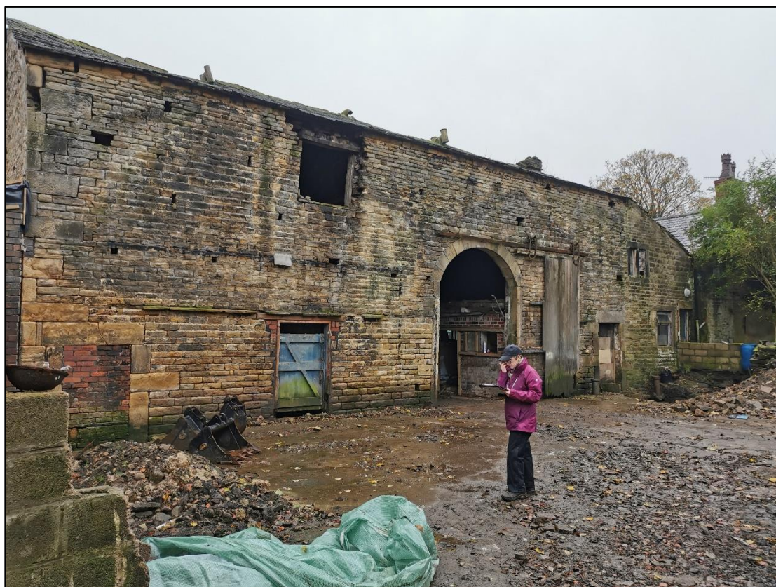
Plate 2 - Barn as viewed from the north looking south view 1
