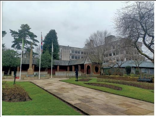
View of the Existing Parkfield House from the Garden of Remembrance
