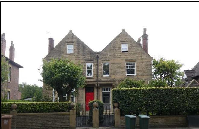
West Lea, 161-163 Manchester Old Road
