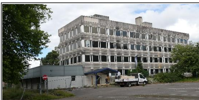
South and East Elevations
