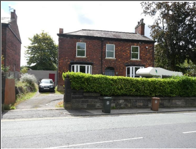
Broomfield, 151 Manchester Old Road
