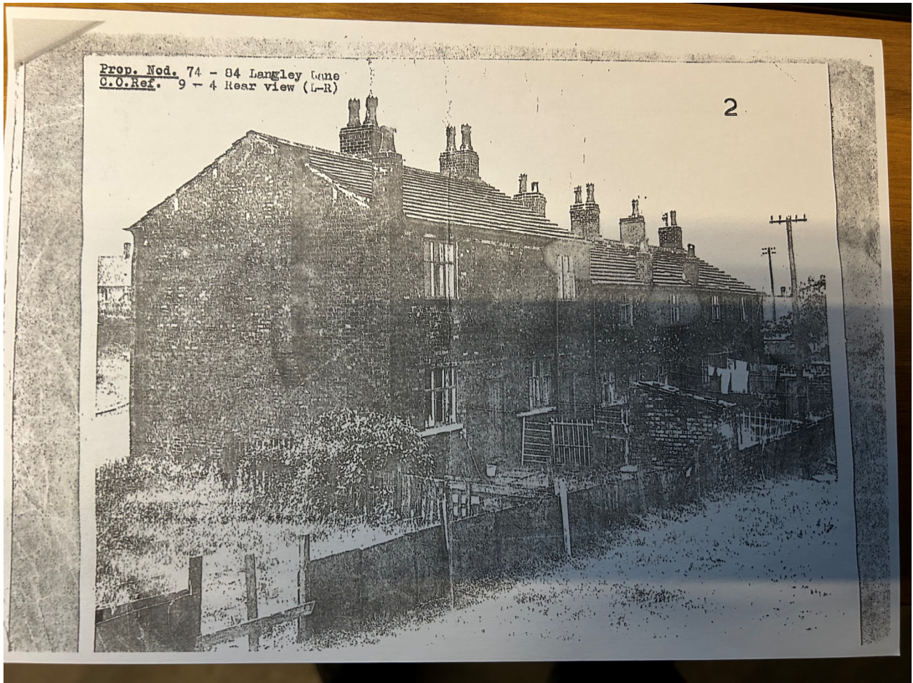
Photo 4: Picture taken of the rear of the Dwellings on site from the north of Langley Lane
