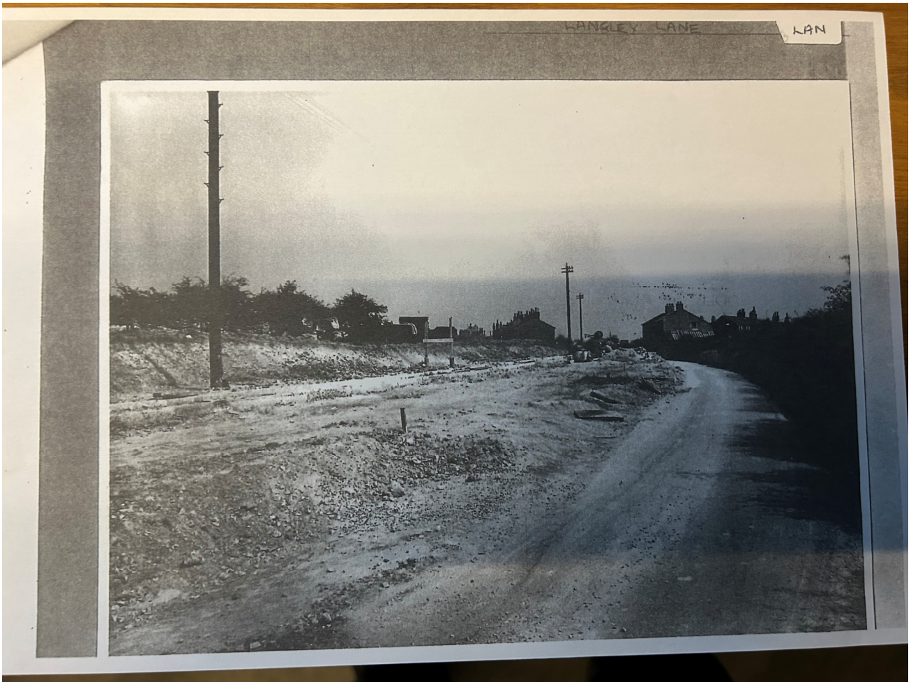
Photo 2 : Picture taken further up the road once dwelling where demolished from the west of Langley Lane
