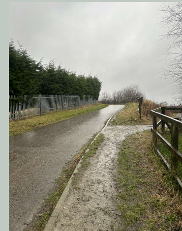
5. View of entrance road.
