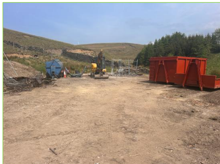
The cleared area
