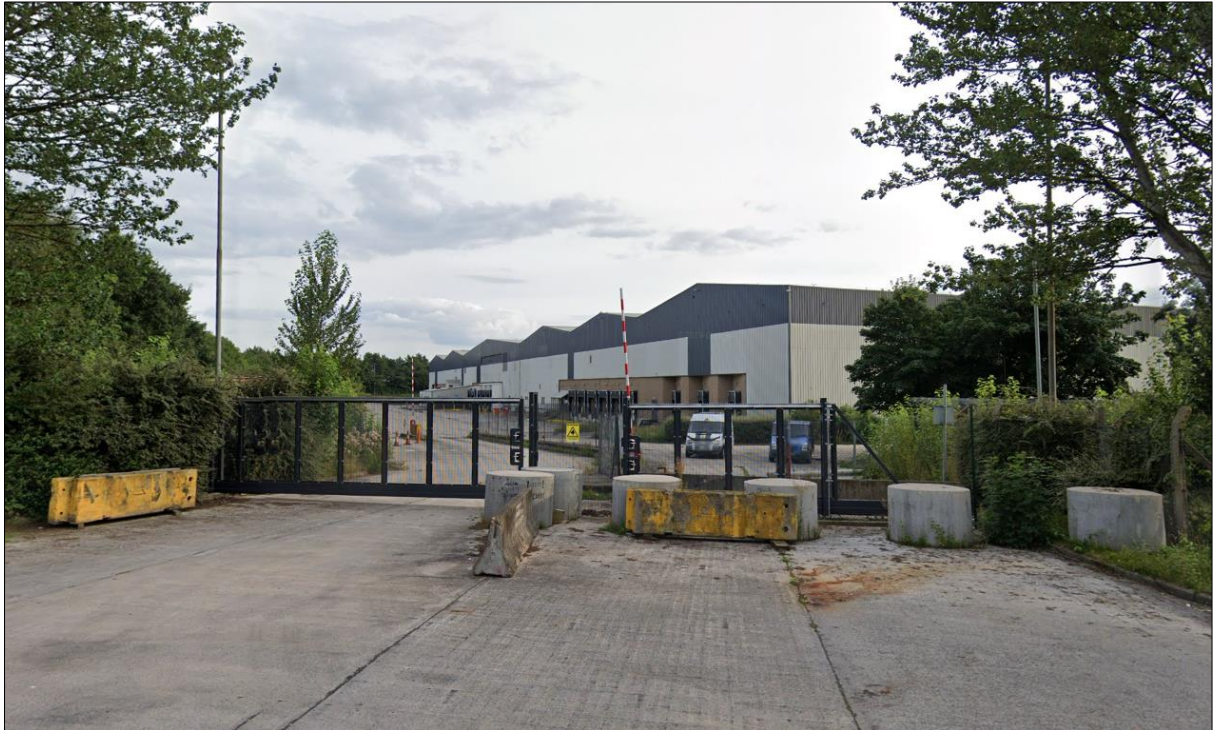
Figure 2: Existing access and warehouse at the Site
