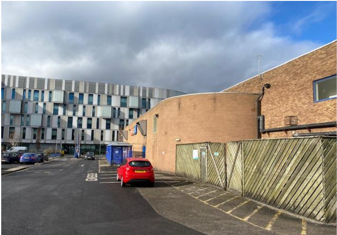
(Figure 6 – Photograph showing the rear elevation of the building and Smith Street car park)
