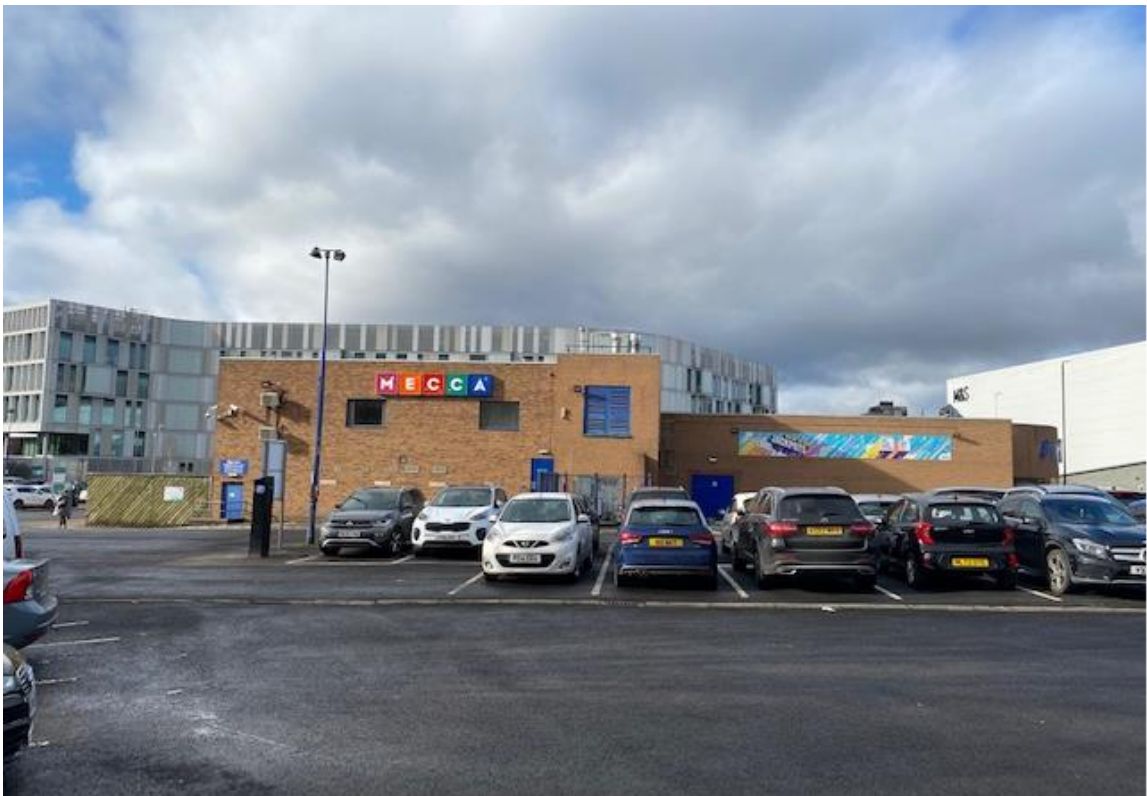
(Figure 5 – Photograph showing the side elevation of the building and Smith Street car park)
