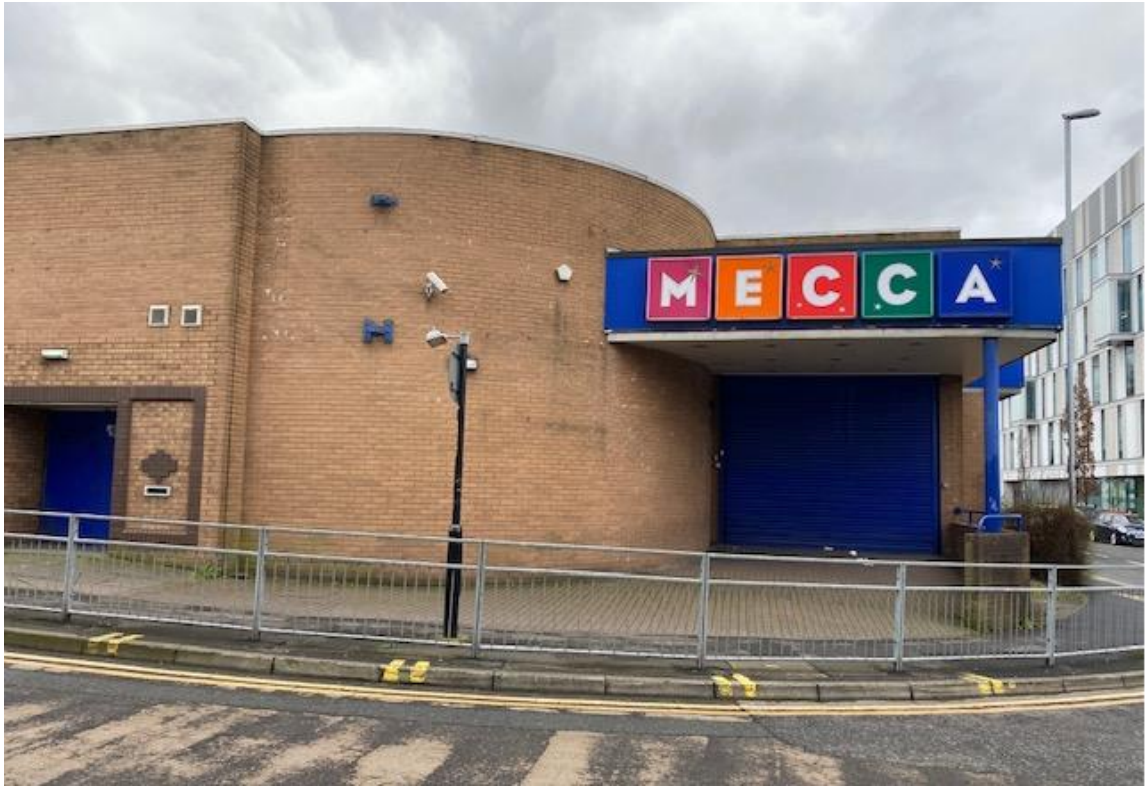
(Figure 4 – Photograph showing the front elevation of the building)
