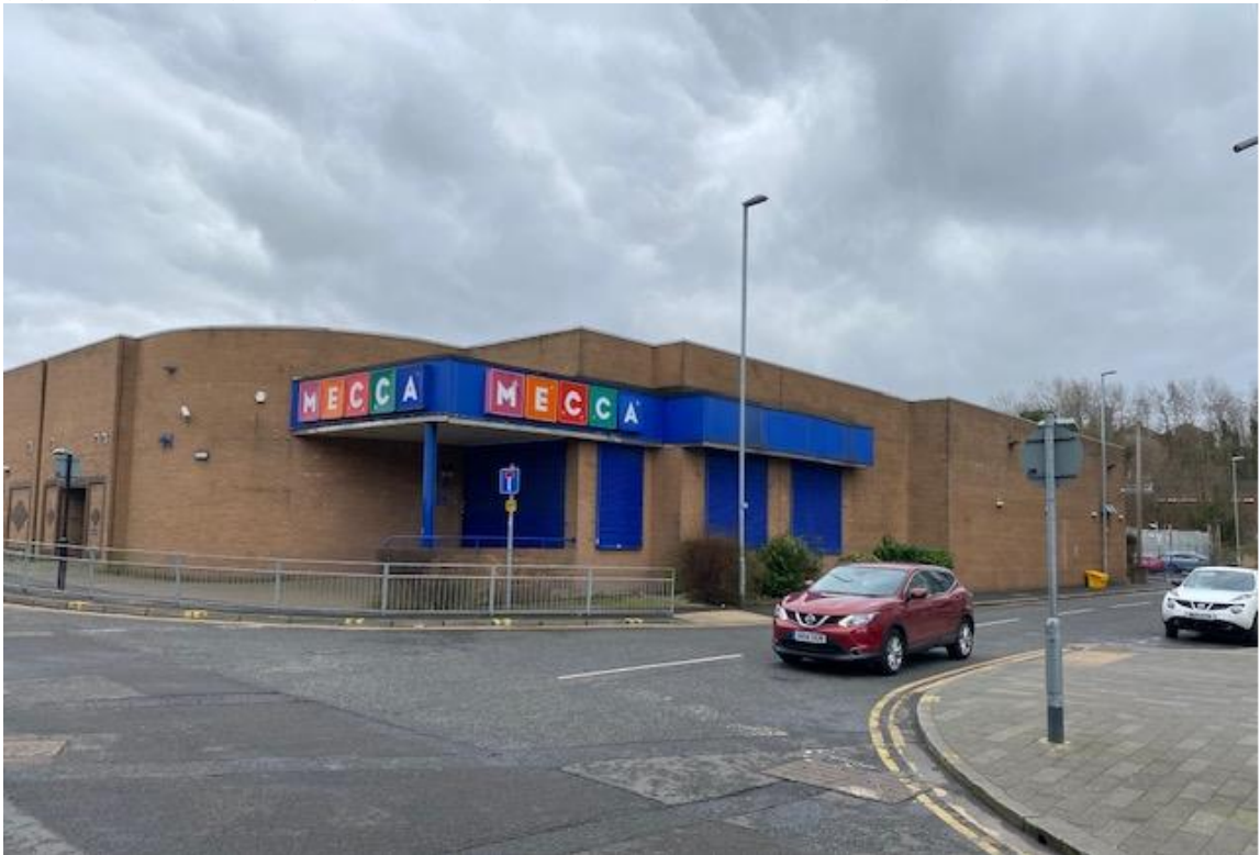
(Figure 3 – Photograph showing the front and side elevations of the building)
