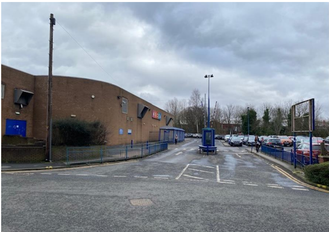
(Figure 7 - Photograph showing the rear elevation of the building and Smith Street car park)
