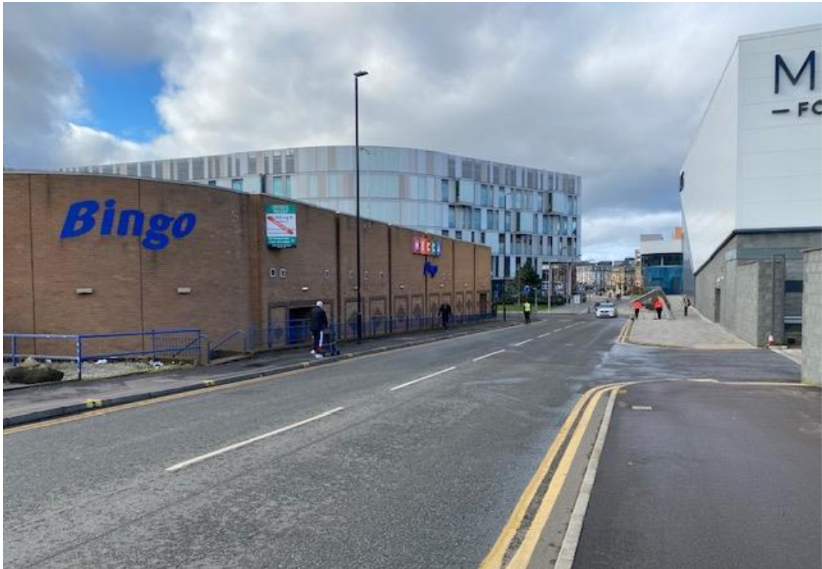
(Figure 8 – Photograph showing the front elevation of the building and wider street scene)
