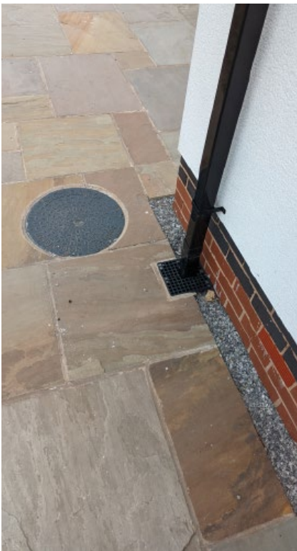
Existing drainage inspection chamber
