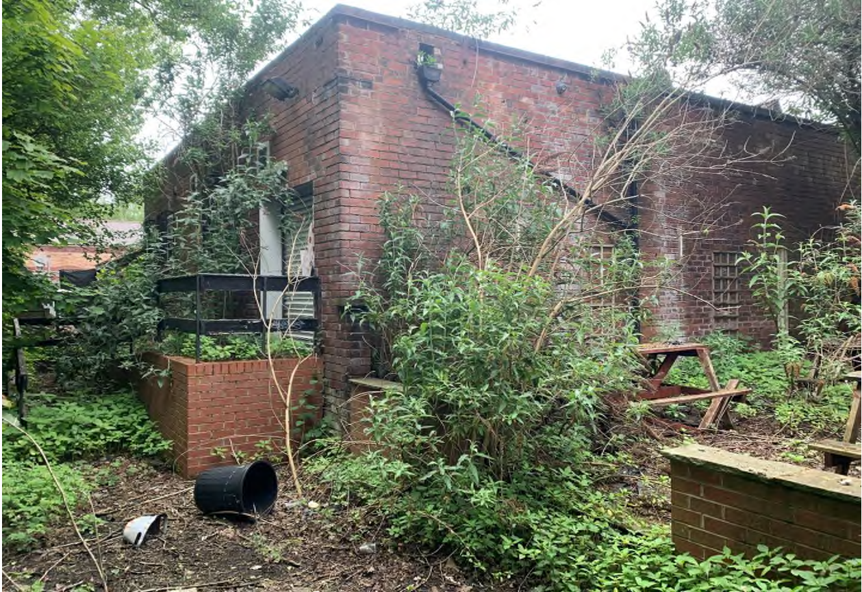
Photograph No 3: View of Outside Space Pre-Demolition
