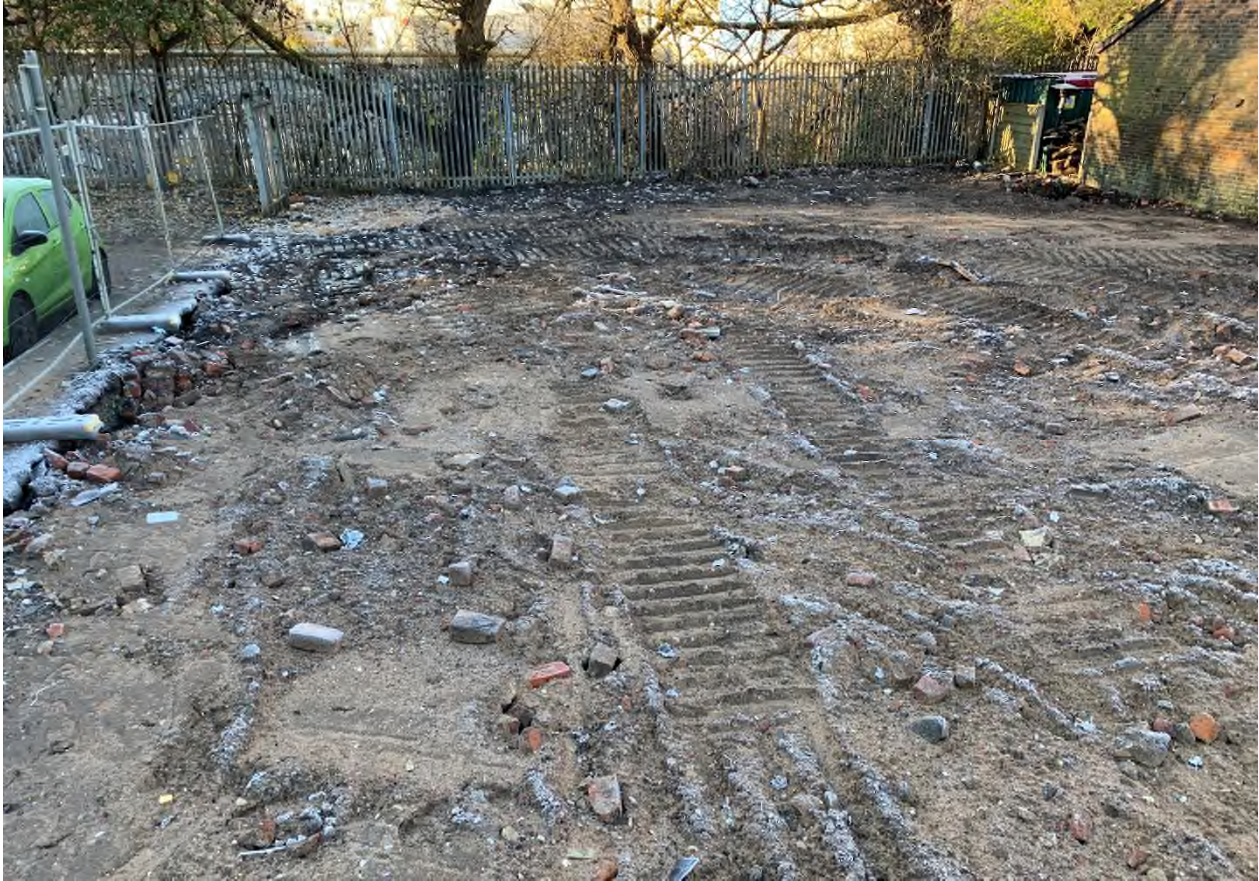
Photograph No 5: View of Site from South-East Corner
