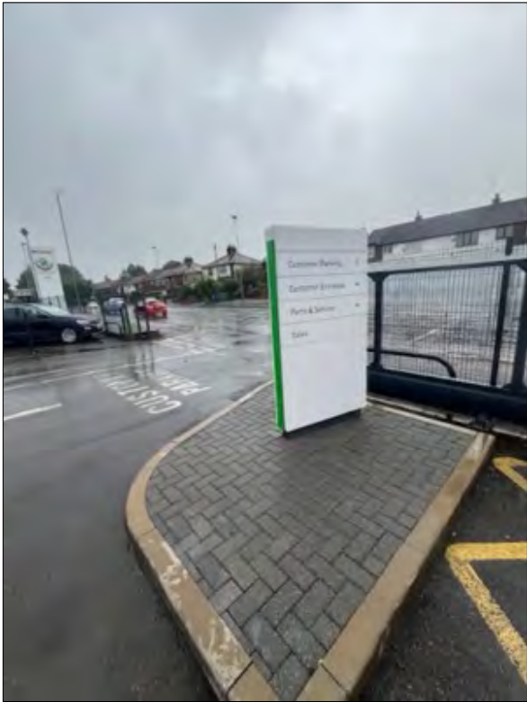
DIRECTIONAL SIGNAGE. GREEN FLASH TO BE WRAPPED OR REPLACED
