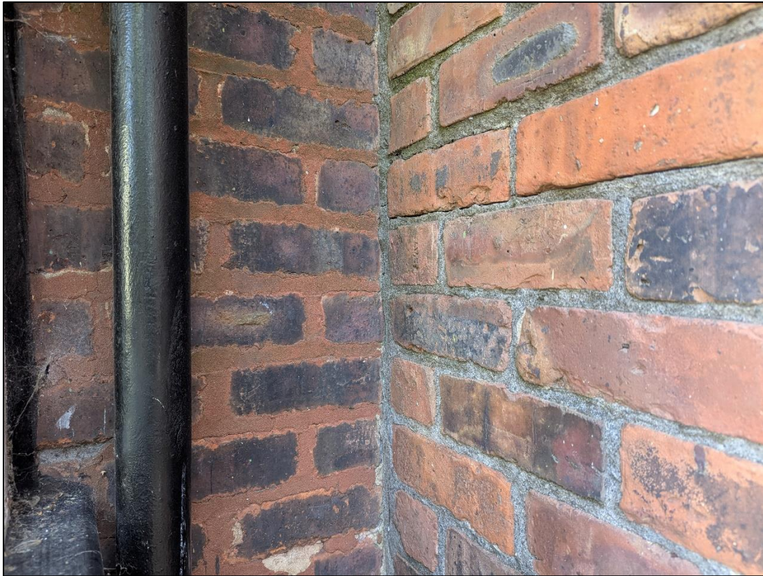
Plate 13: Brickwork of extension (right) butting against house (left)
