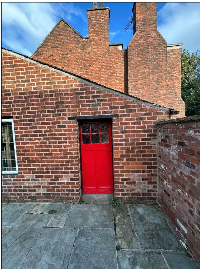
Plate 6: External doorway to garage to be converted to window
