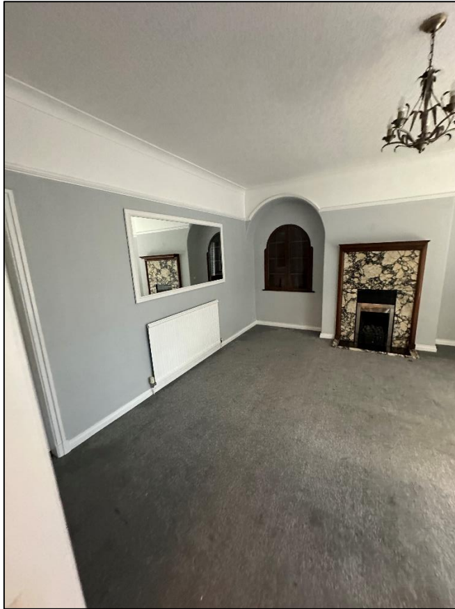
Plate 5: Interior arched opening to blocked window with cupboard inserted
