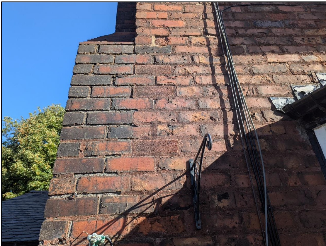
Plate 10: Comparison of brickwork of stack and house
