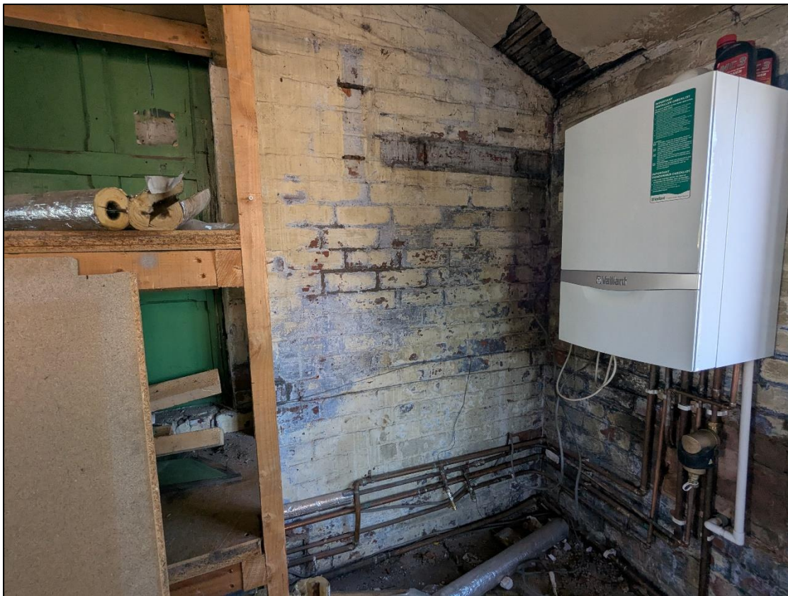
Plate 4: Northwest corner of garage
