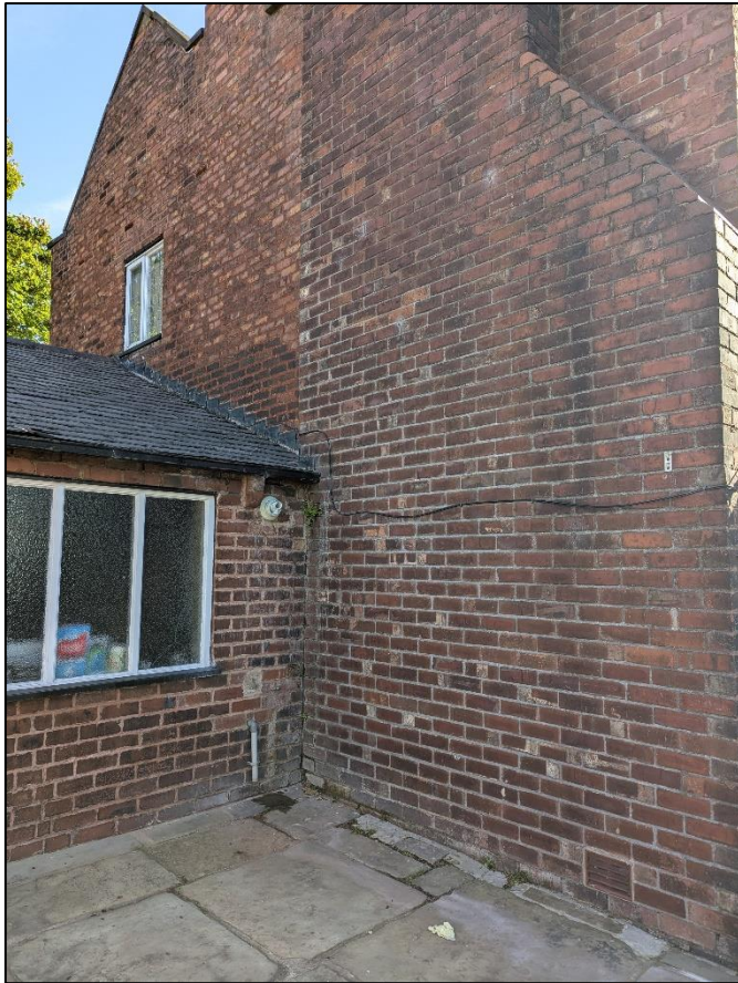
Plate 9: Detail of brickwork to external stack
