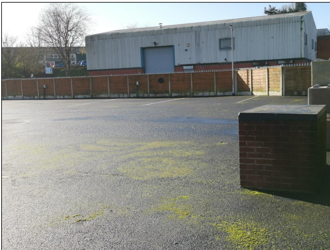
Figure 1 – View to south boundary.
