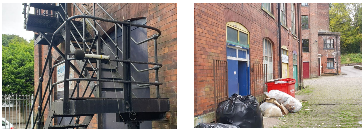
Figure 4: Site Location Measurement Pictures
