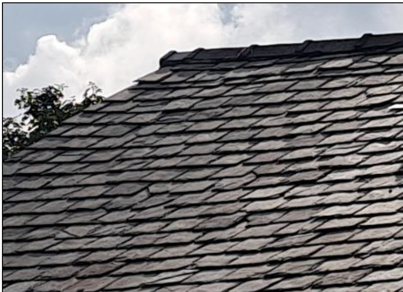
Photograph 10 showing a section the roof
