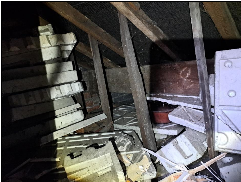
Photograph 13 showing a section of the roof void
