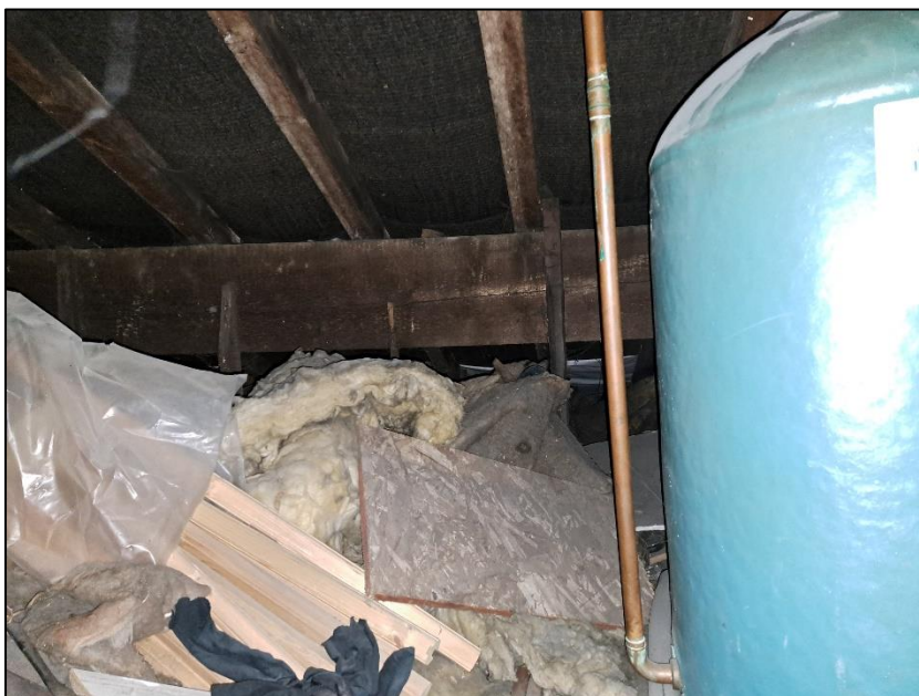
Photograph 14 showing a section of the roof void
