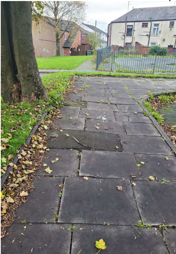
Root disturbance to paving from T2
