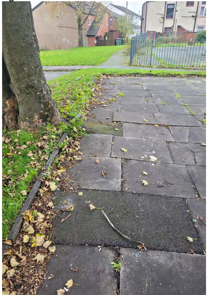
Root disturbance to paving from T2
