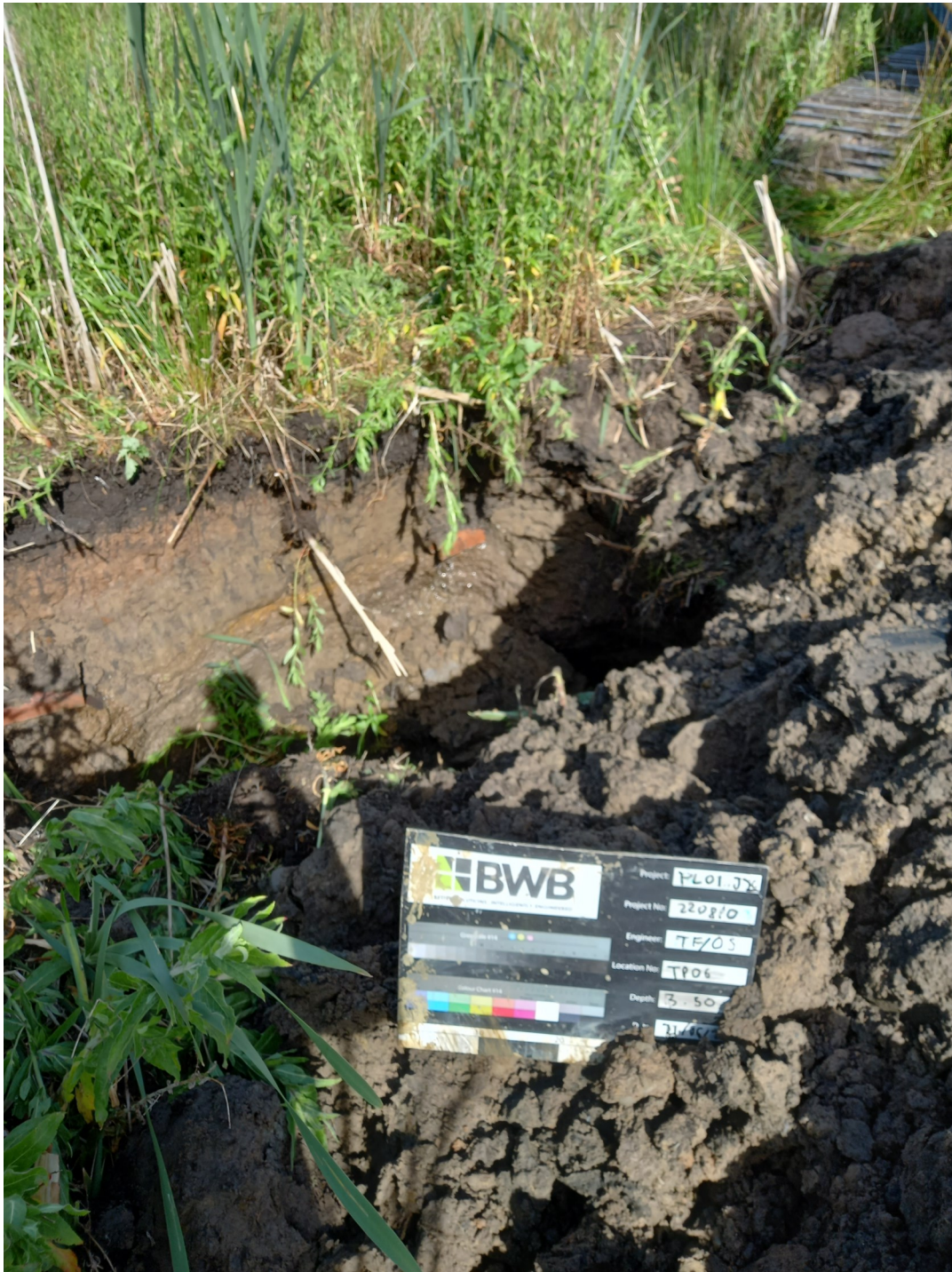
Photo 2: TP06, with land drain visible in pit wall
