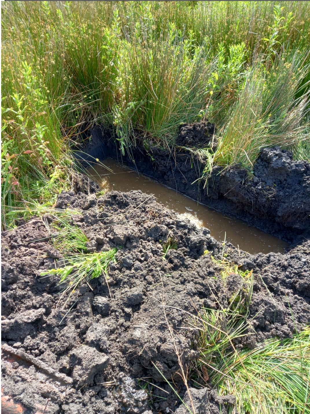
Photo 2: TP05, infilled with water due to land drain
