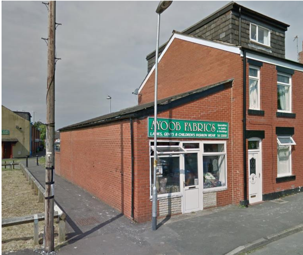
Above: Front elevation of existing single storey building.
