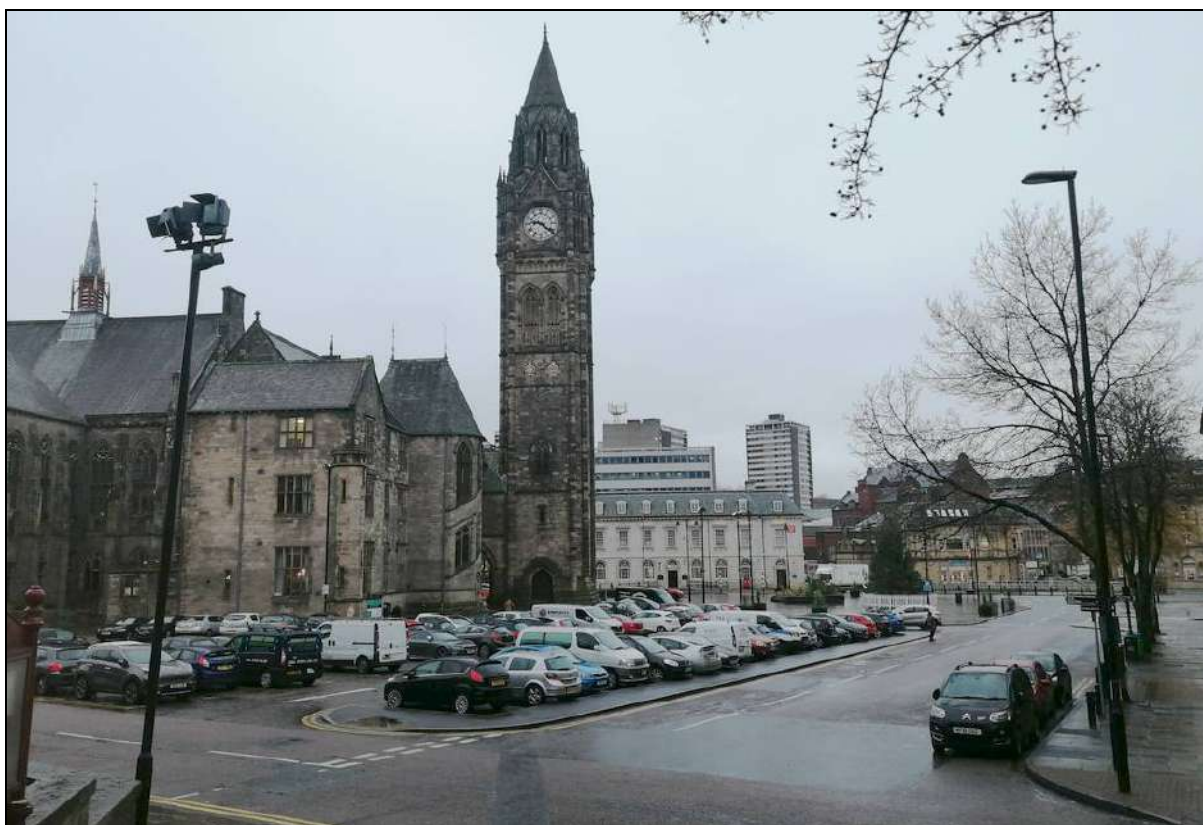
Plate 5: View north along Packer Street and the car-parking areas that dominate Town Hall Square
