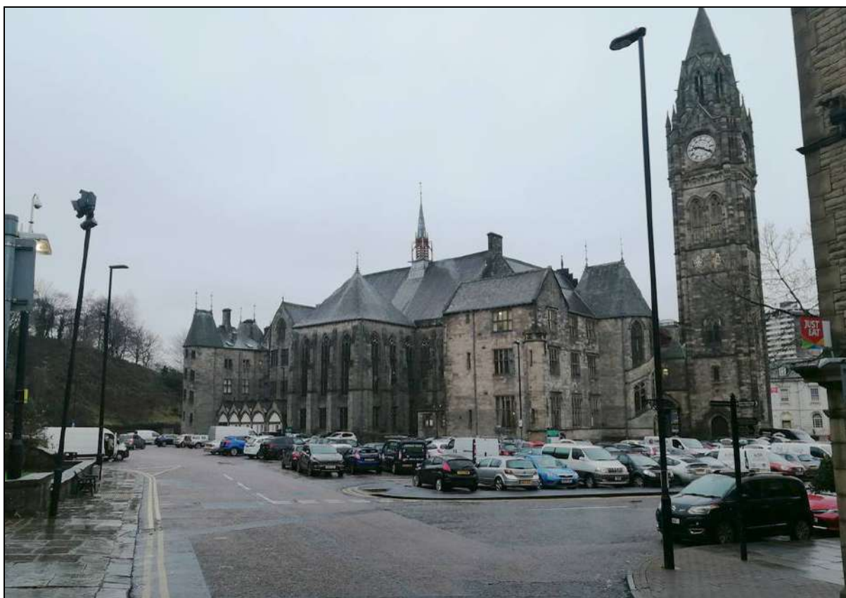
Plate 6: View west across the car-parking area to the rear of the Town Hall
