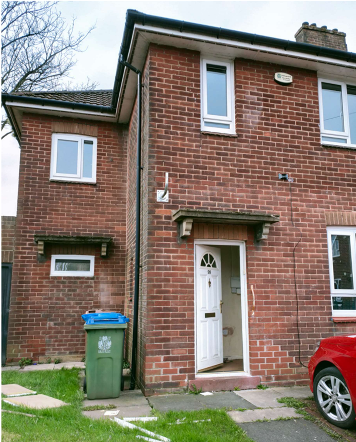
Above – view showing extant front door to right, and sealed access to left
