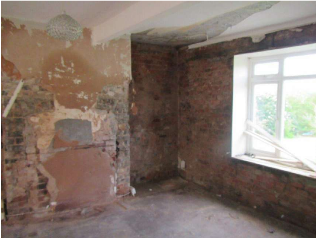
Photograph 17 – Example of internal conditions within Building 1.
