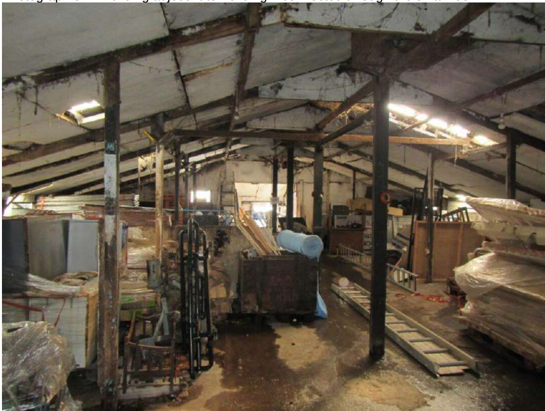
Photograph 32 – Interior conditions within Building 10.
