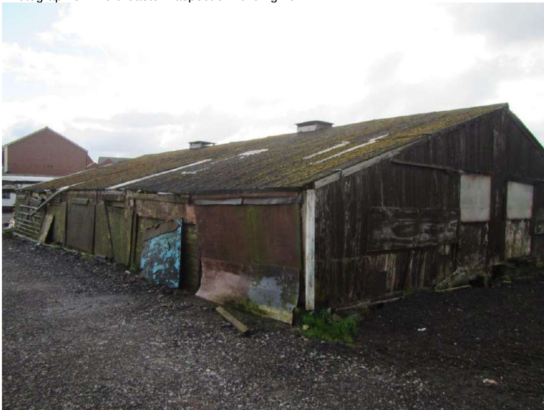
Photograph 6 – Southwestern aspect of Building 10.
