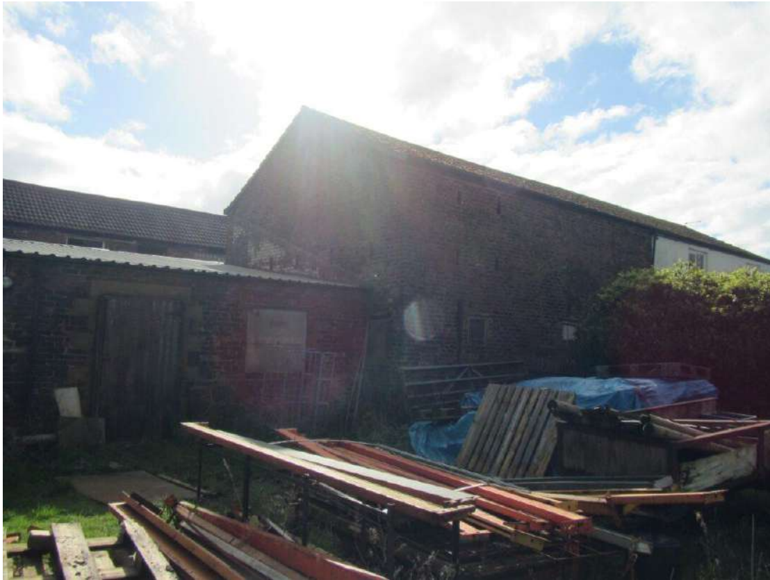
Photograph 3 – Southern aspects of Buildings 1 & 2.
