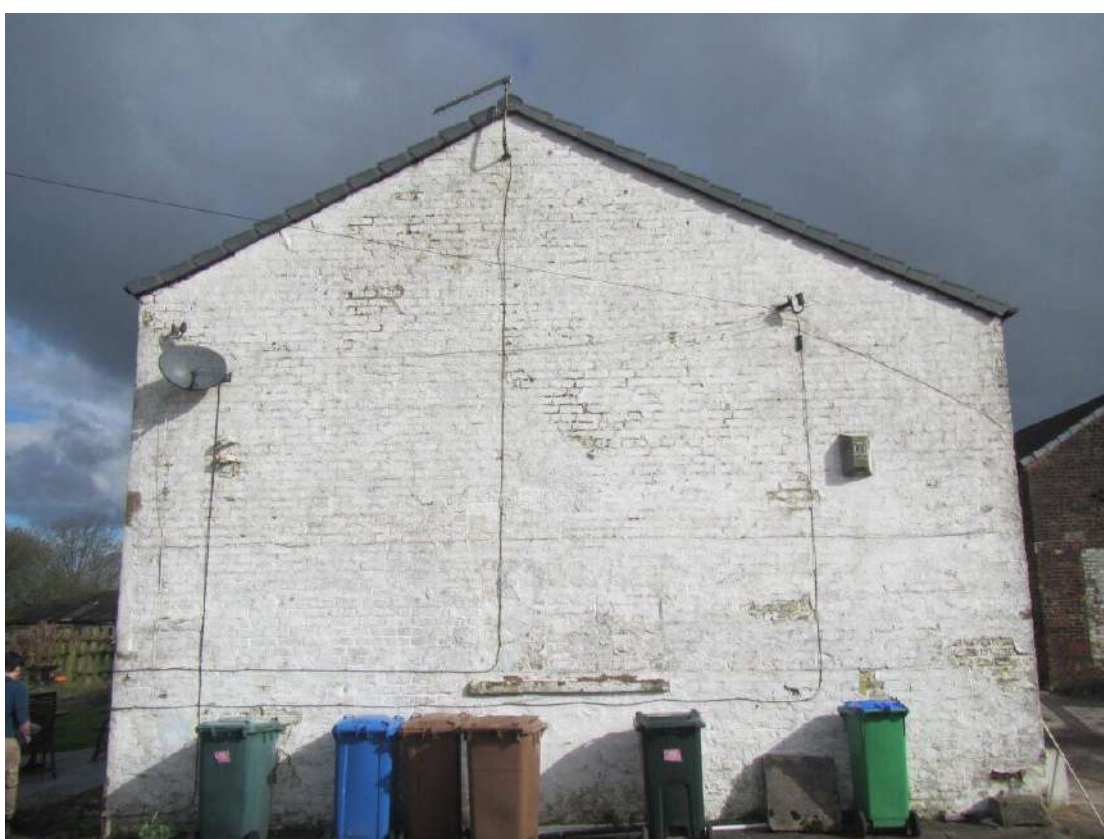
Photograph 2 – Eastern aspect of Building 1.
