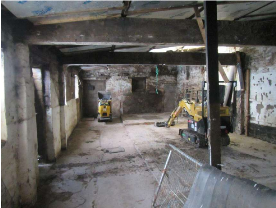
Photograph 31 – Building adjacent to Building 2 connected through the small room.
