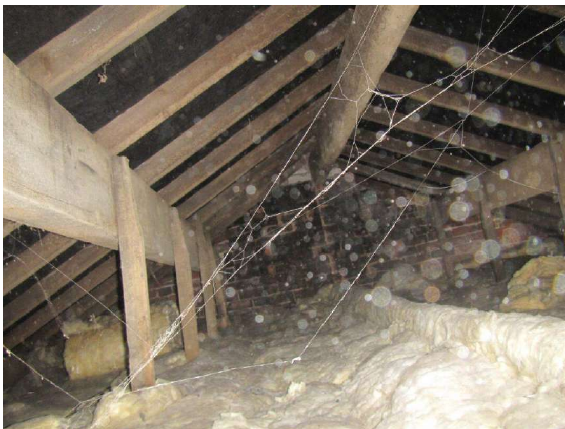
Photograph 21 – Eastern end of roof void of Building 1 (past the internal wall).
