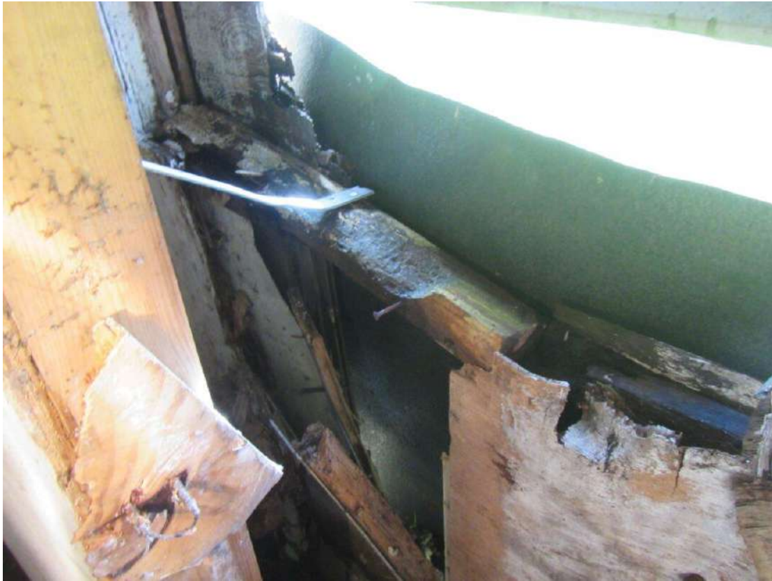
Photograph 33 – Wall structure and cavities in Building 10.
