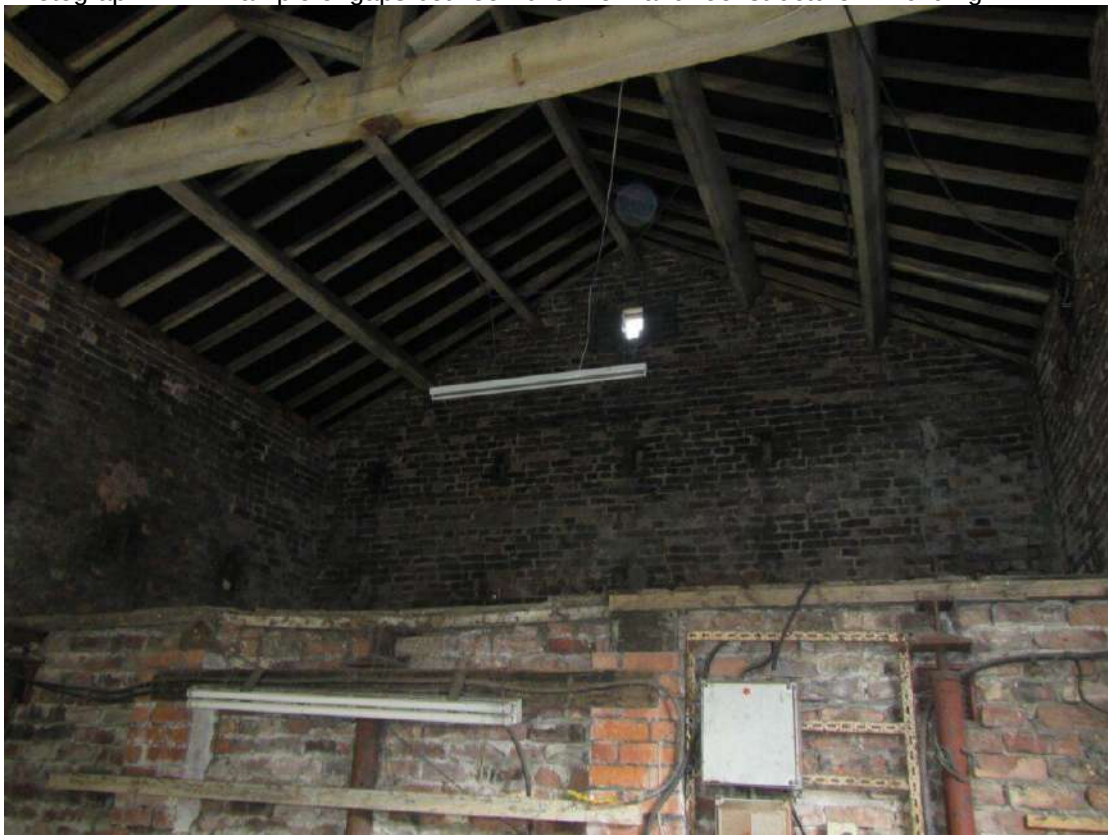
Photograph 28 – Small room created by internal wall on eastern end of Building 2.
