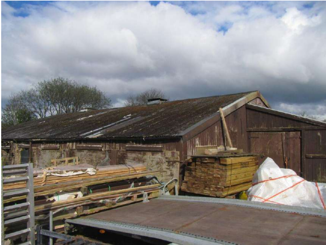
Photograph 5 – Northeastern aspect of Building 10.
