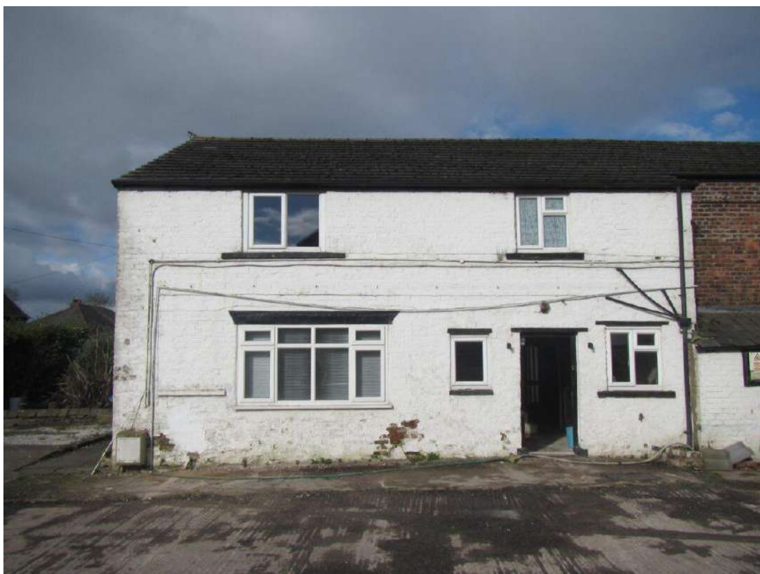
Photograph 1 – Northern aspect of Building 1.
