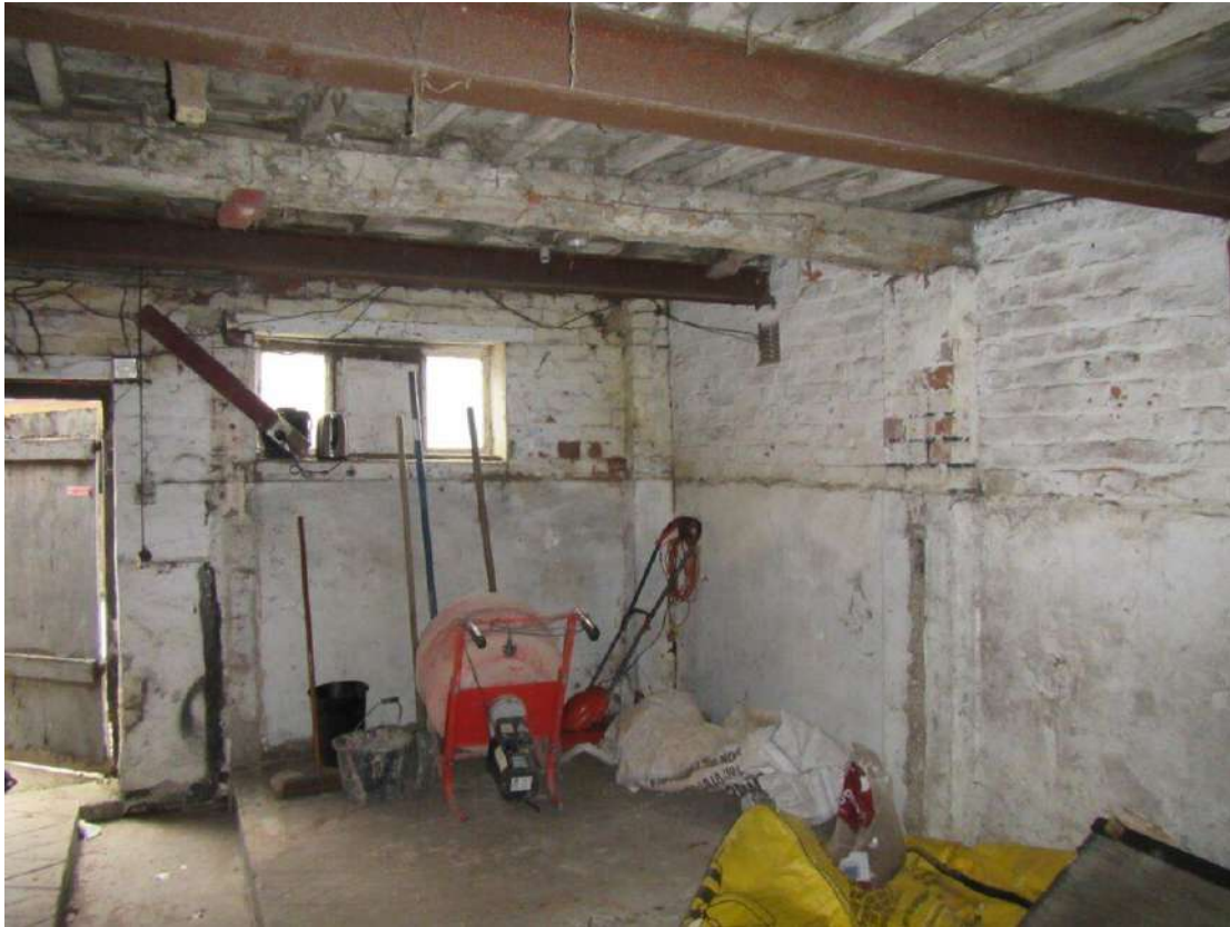
Photograph 29 – Small room on eastern end of Building 2.
