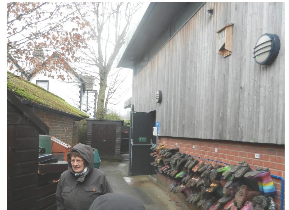
Timber cladding used to the North East of the site
