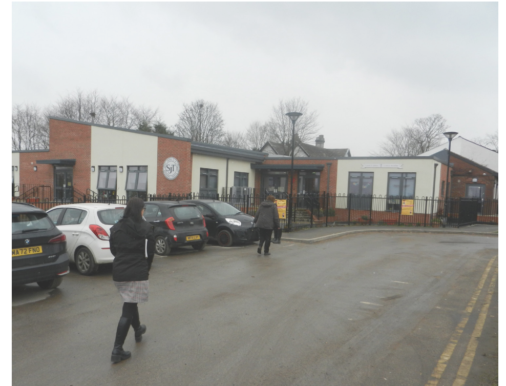
View of the school from the car park
