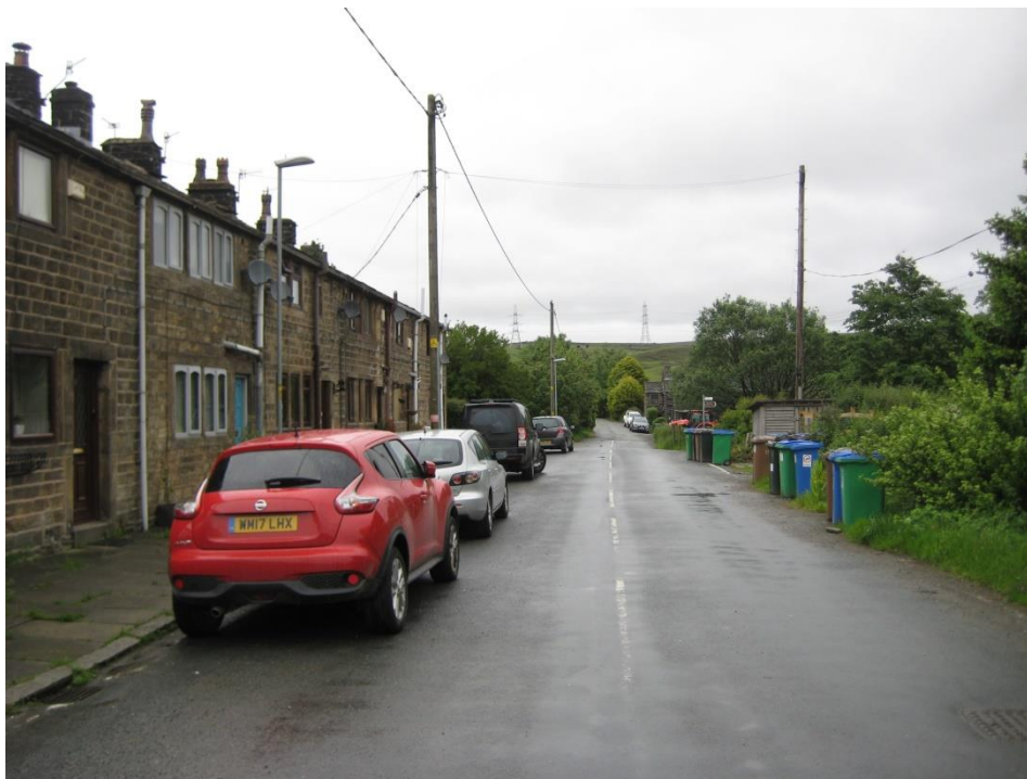
Figure 11: Frontage of 9-19 Salley Street viewed from front Salley Street
