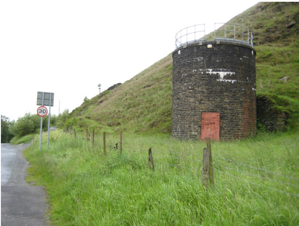
Figure 10: Summit Tunnel Ventilation shaft to the north of Salley Street.
