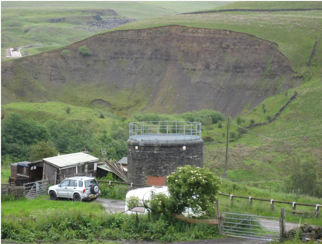
Figure 9: Summit Tunnel Ventilation shaft to the southeast of the application site.
