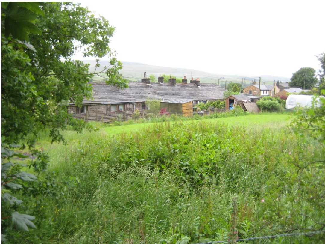
Figure 14: View of the rear of 9-19 Salley Street
