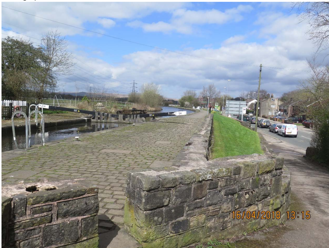
View up to locks 54, viewing away from site along Bentley Avenue
