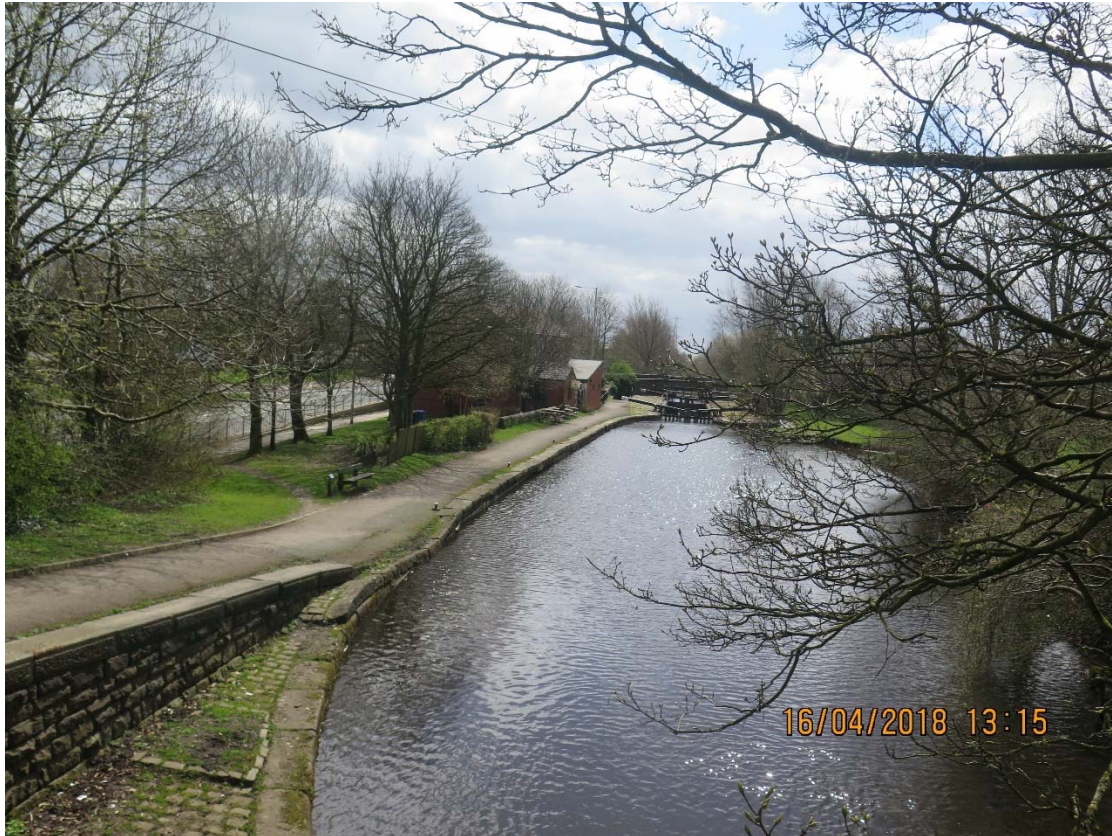
View down to bottom locks tunnelling under Rochdale Road
