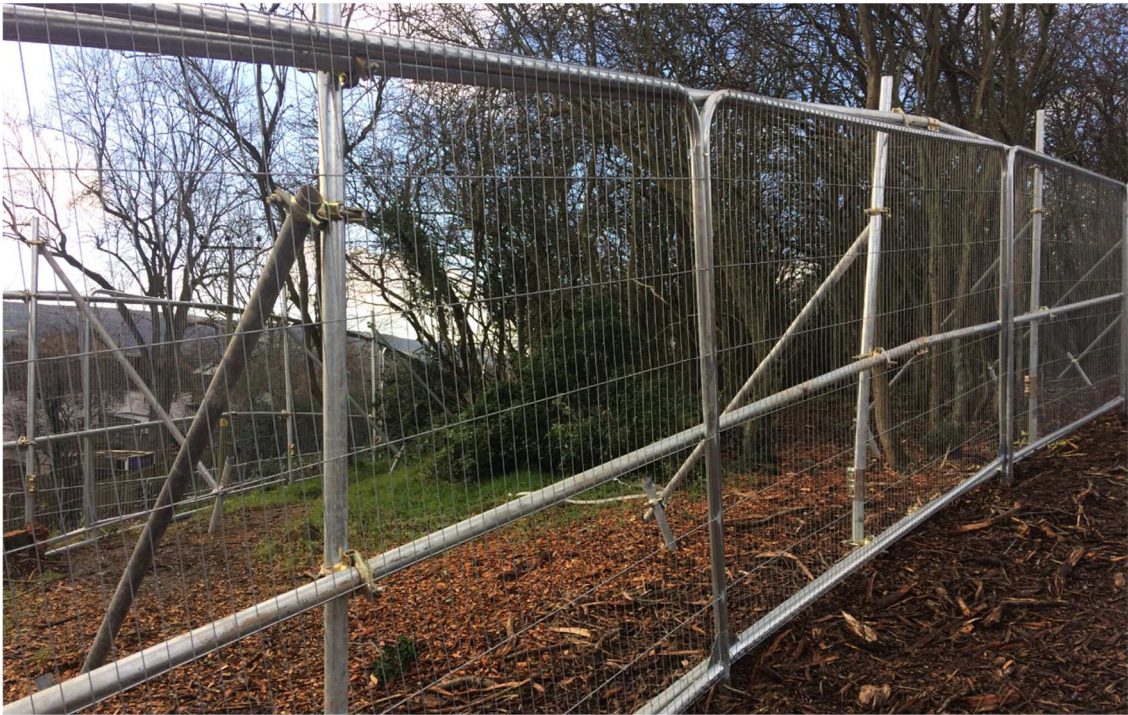
Above: Full specification barrier fencing.
