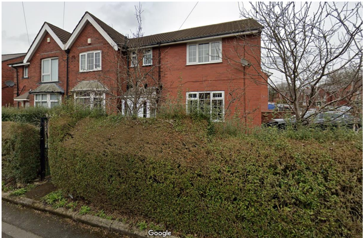
Similar Extension at 110 Edmund Street
