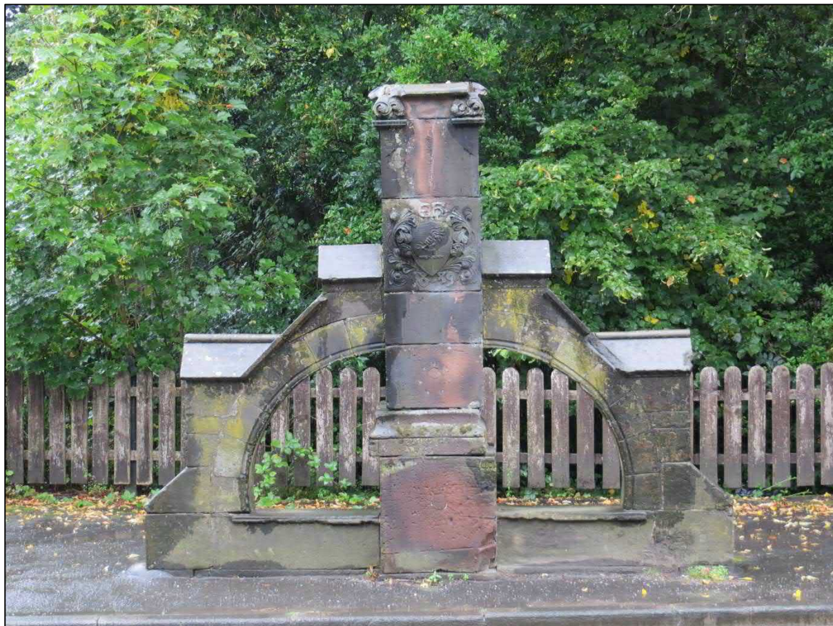
Figure 37: View of Fountain Horse Trough to North of White Hart Inn looking west. September 2019
