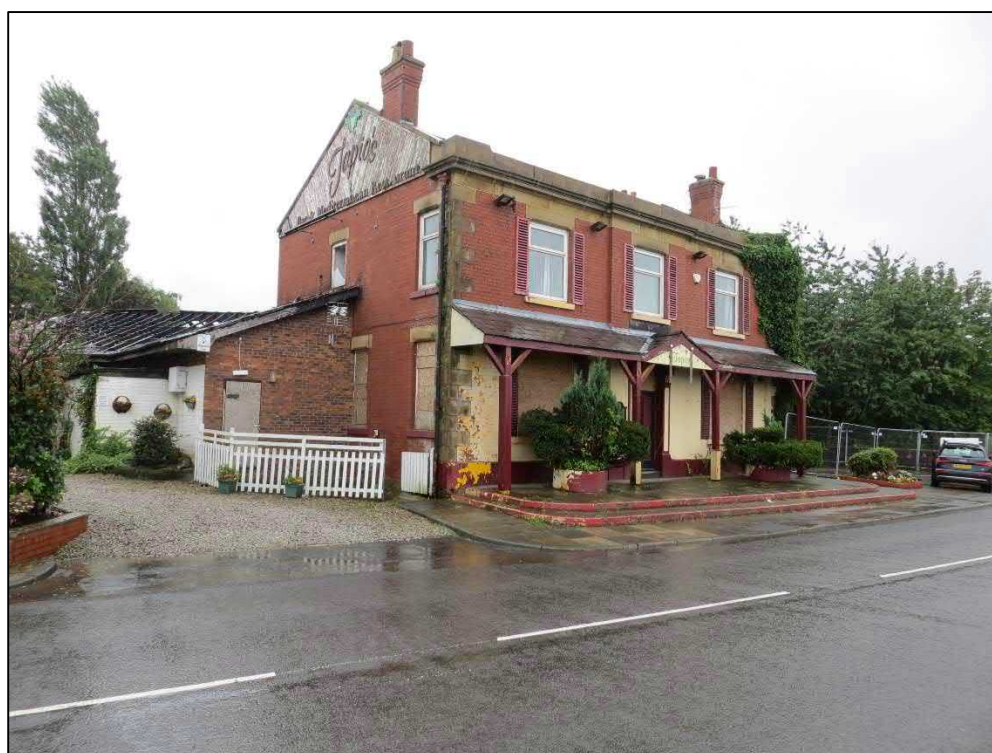
Figure 18: Photograph of former “Tapio’s” restaurant September 2019.
