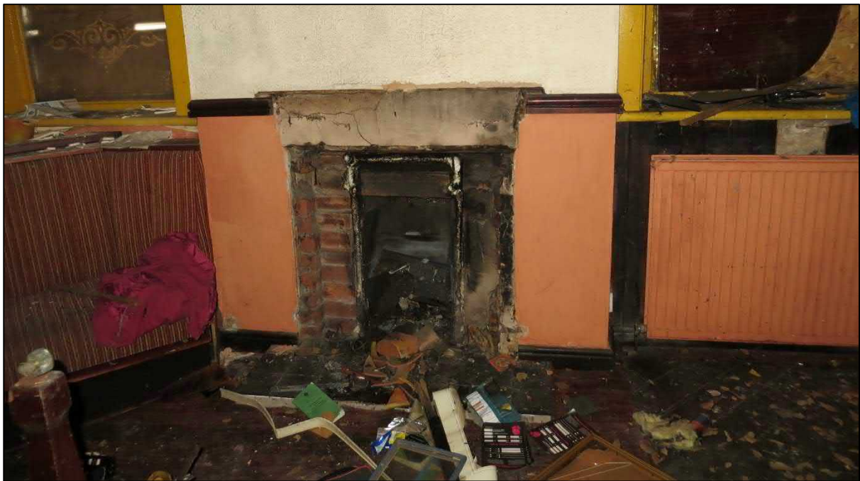
Figure 28: All original ground floor interior features have been removed.
