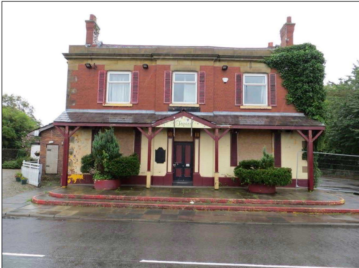
Figure 19: Front (east) elevation.
