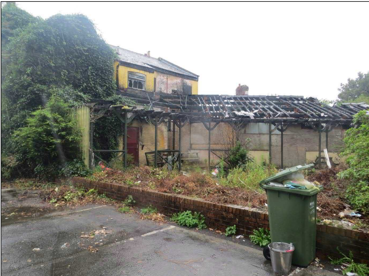
Figure 23: Rear (east) elevation and extension.
