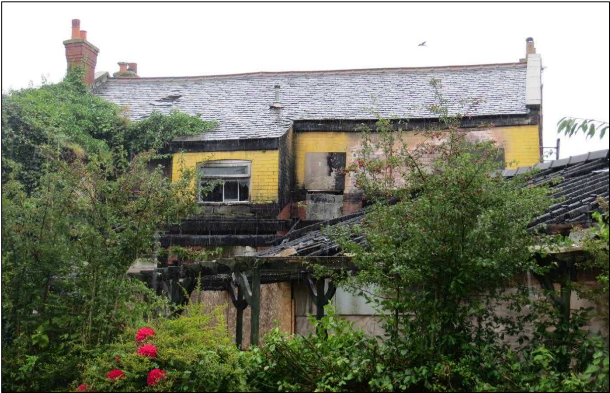
Figure 24: Rear (east) elevation and extension.
