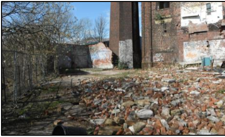
Demolished extension to S side of original mill building & demolished Building 8 in b/g. Area previously noted as being used for drum/IBC storage.
