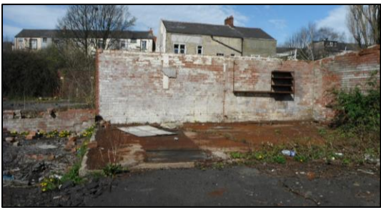
Storage/Service (Building 3 to N of Site).
