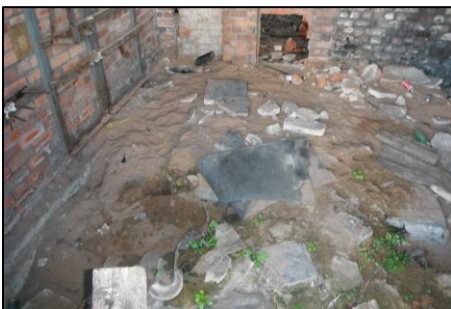
Former substation outbuilding.
