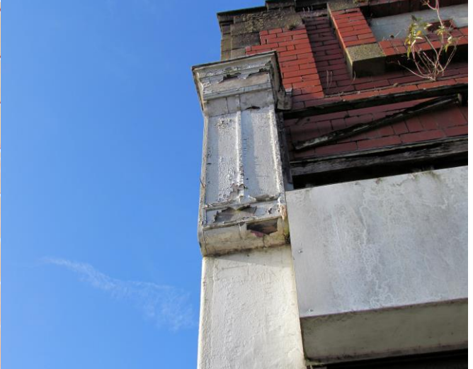
Detail of Console (Photo no. 8)
