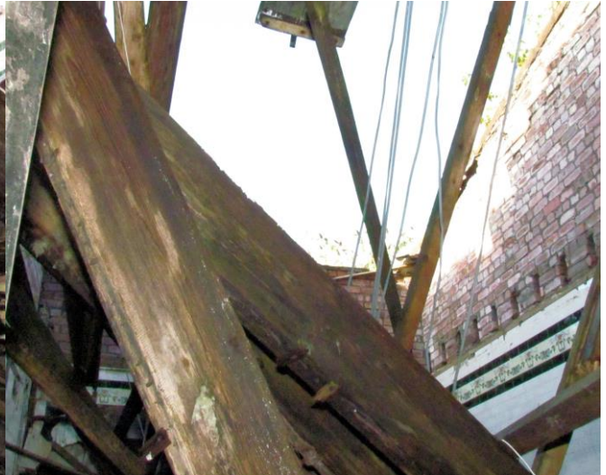
View Into Number 44 Showing Party Wall with Number 38 (Photo no. 32)
