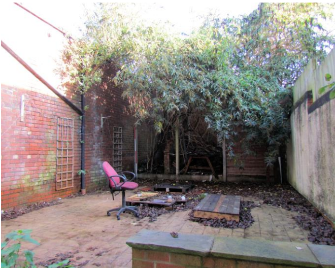
Rear Elevation of Number 44 (Photo no. 13)
