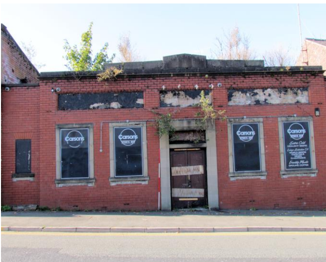
Front Elevation of Number 38 (Photo no. 3)
