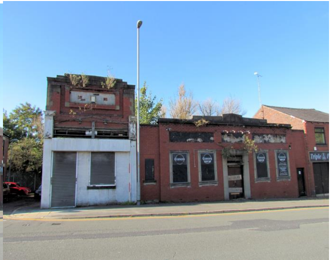
Front Elevation of both Buildings (Photo no. 2)
