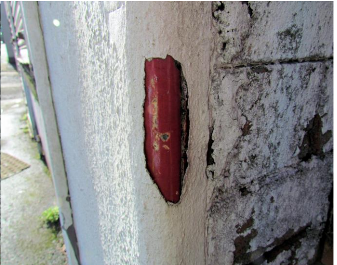
Detail of Evidence of Tiling (Photo no. 10)
