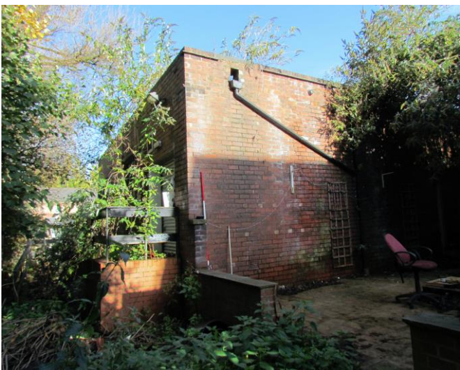
View of West Rear Elevation of Number 38 (Photo no. 15)
