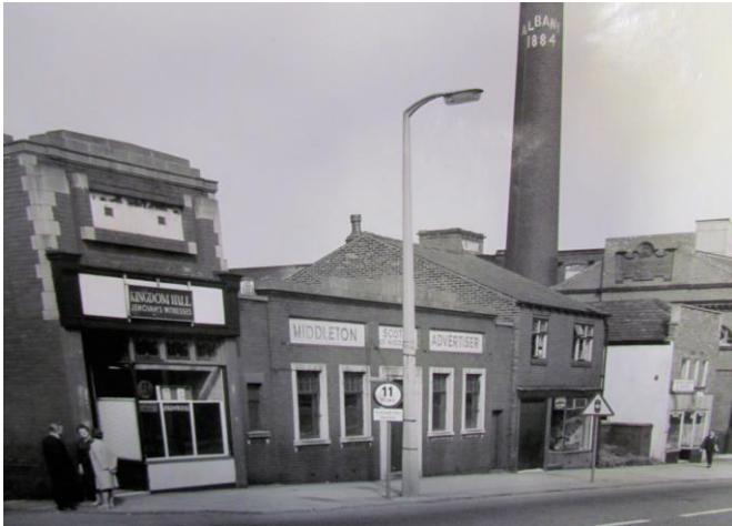
38-44 Townley Street Front Elevation, 1967, by L. Kaye (Middleton Library, ref. E27)
