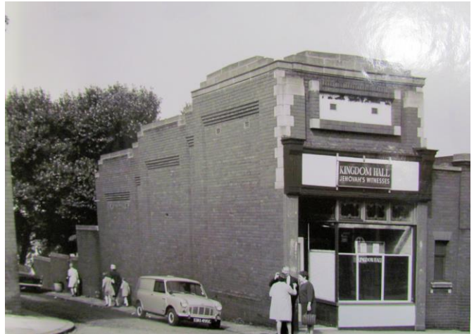
38-44 Townley Street South Elevation, 1967, by L. Kaye (Middleton Library, ref. E27)
