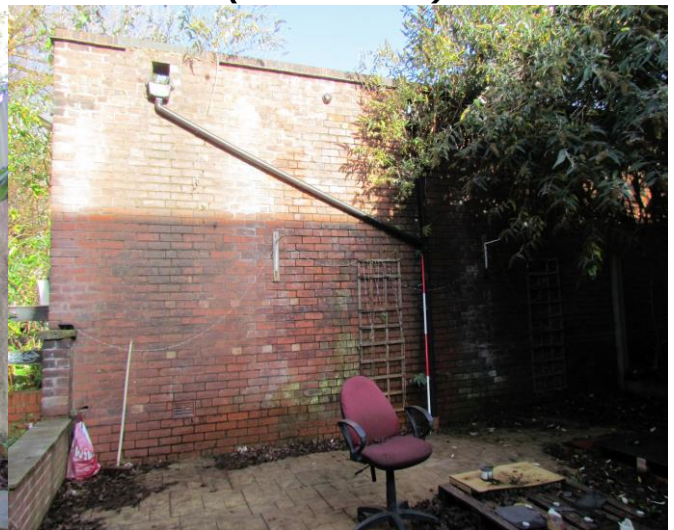
South Elevation of Number 38 (Photo no. 14)
