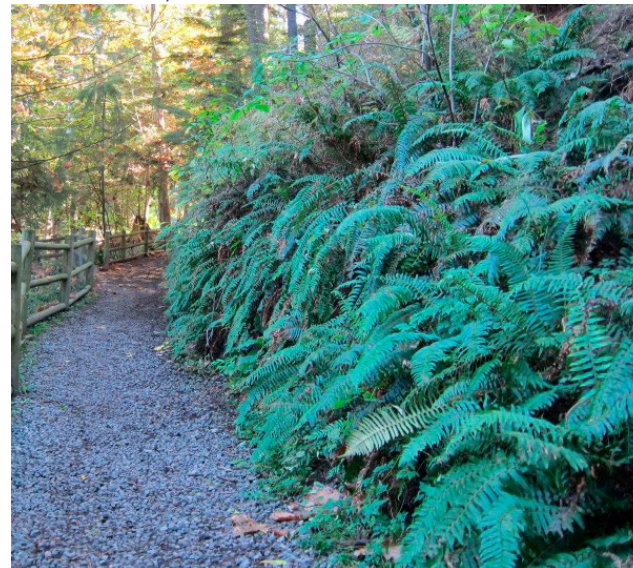
Flex MSE once planting is well established
