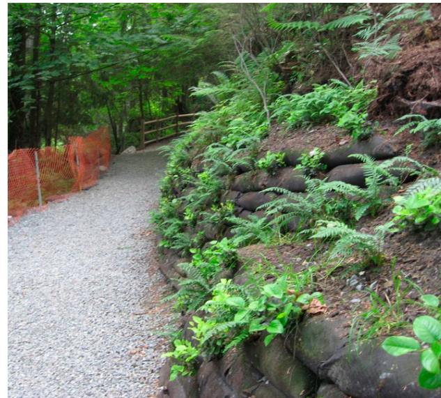
Flex MSE shortly after construction
