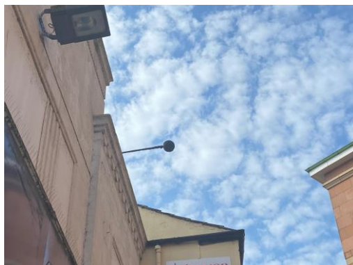
Monitoring above first floor position 2
