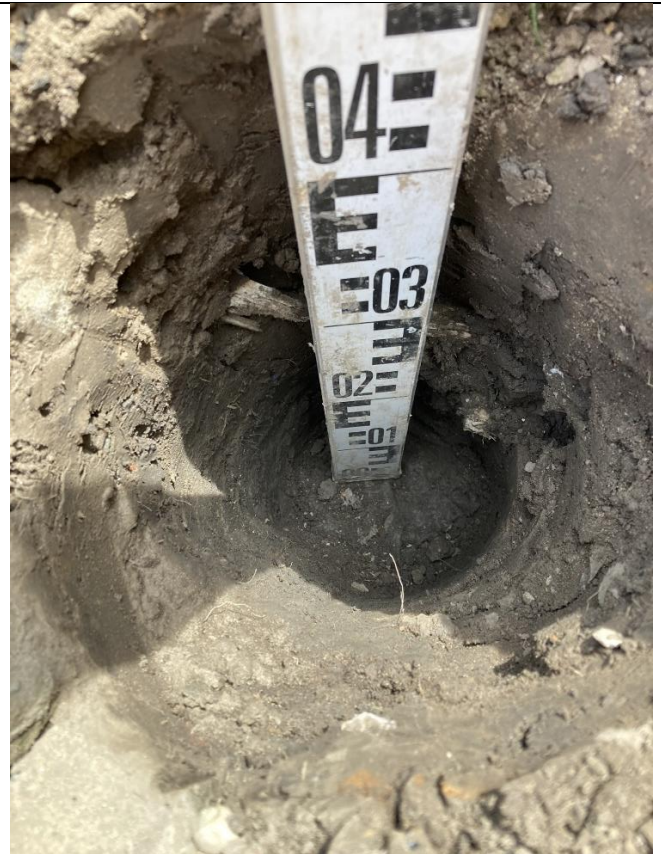
Plot 85: Internal View of excavation
