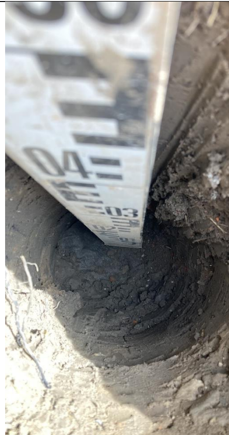
Plot 82: Internal View of excavation
