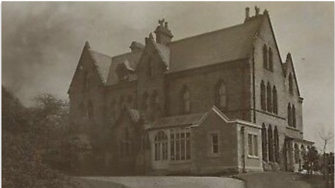
View of the original house from the south west showing the original gable at the north west corner and the glazed structure at ground floor level
