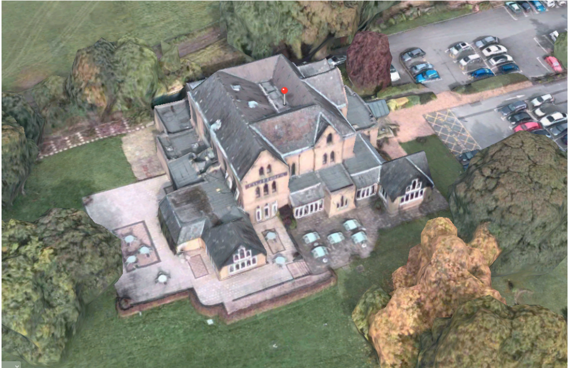
View of current arrangement of ground floor extensions
