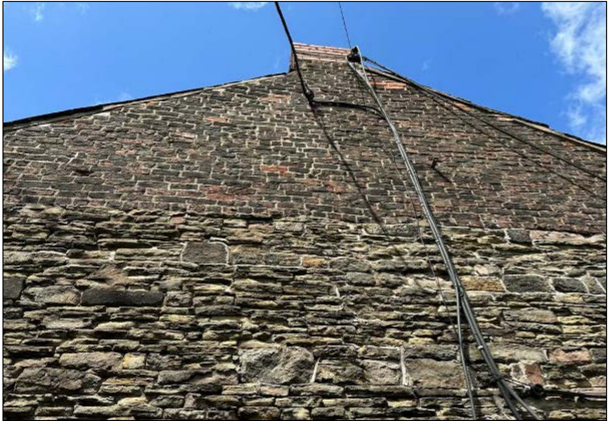
7. Stone and brick above on the southeast elevation
