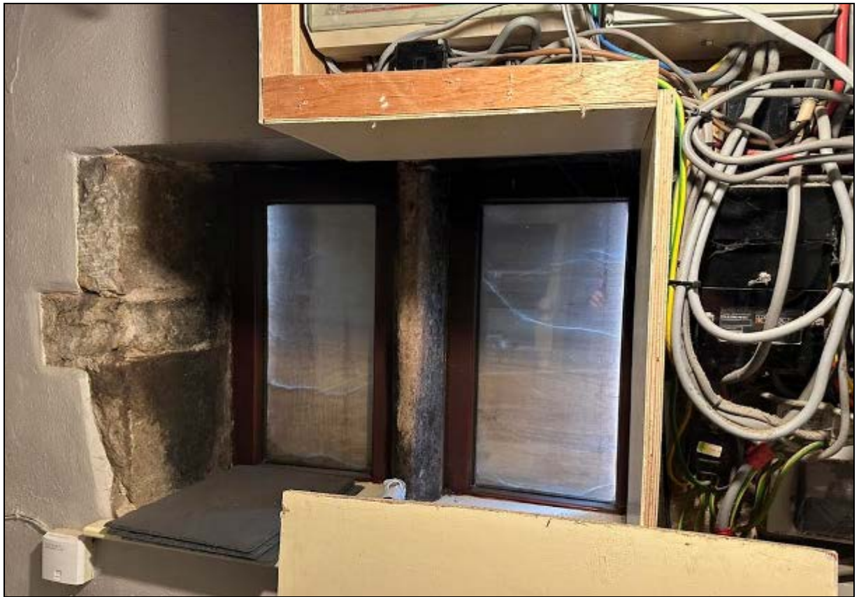
12. Two-light window at foot of staircase
