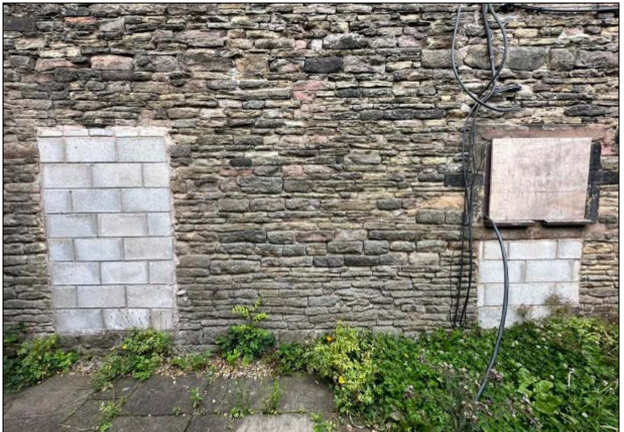
8. Blockwork on southeast elevation and boarded two-light window
