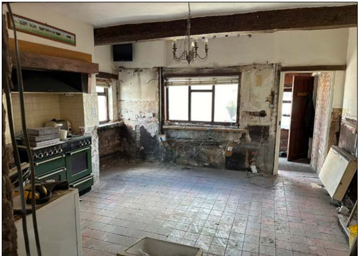
11. The kitchen, with reused beams
