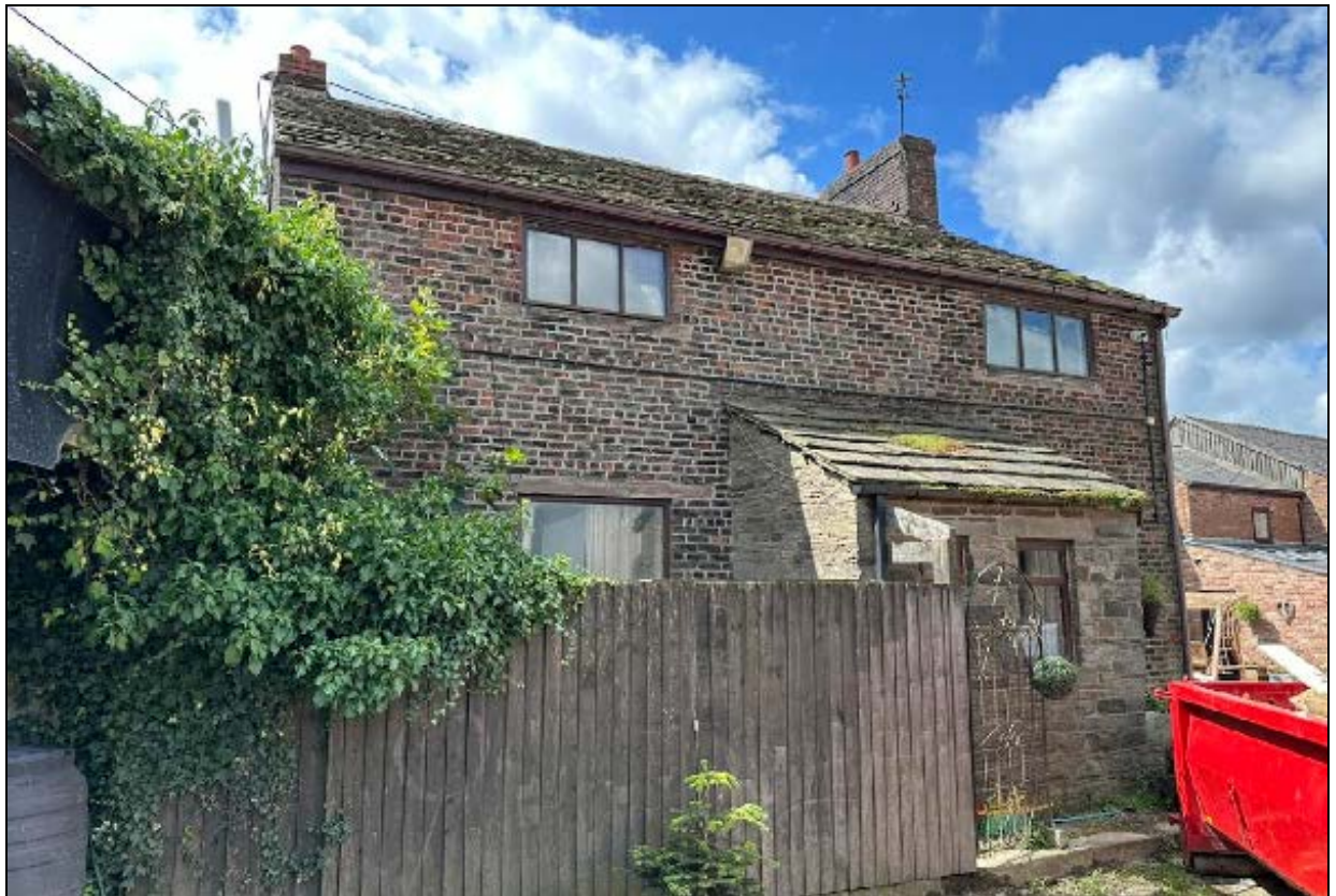
4. Rear elevation, with later stone porch
