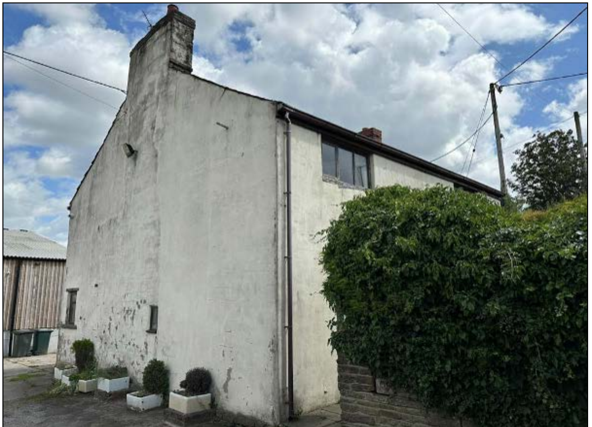
6. The northwest elevation
