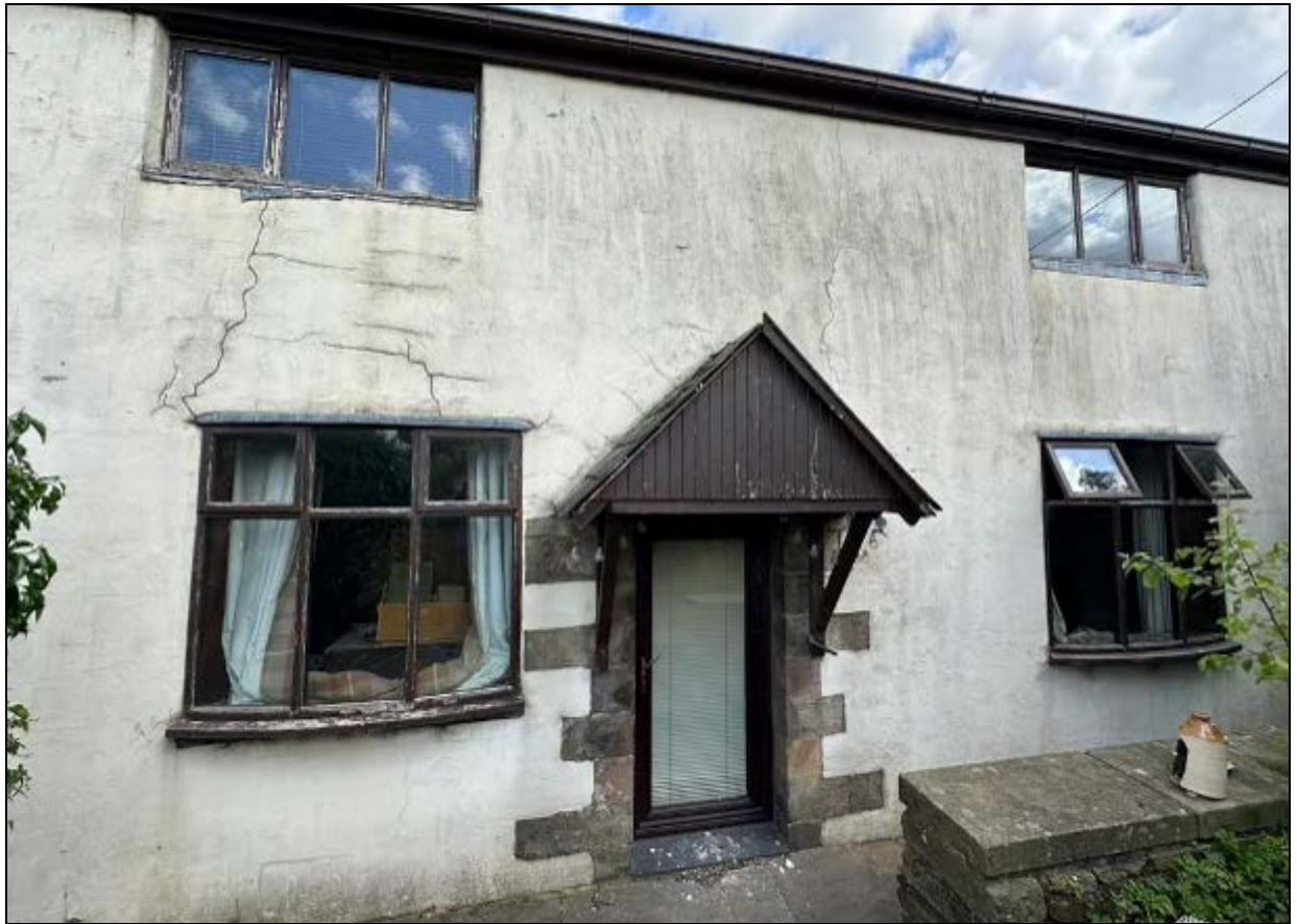
3. The door surrounds is the only visible historic feature in the altered front elevation
