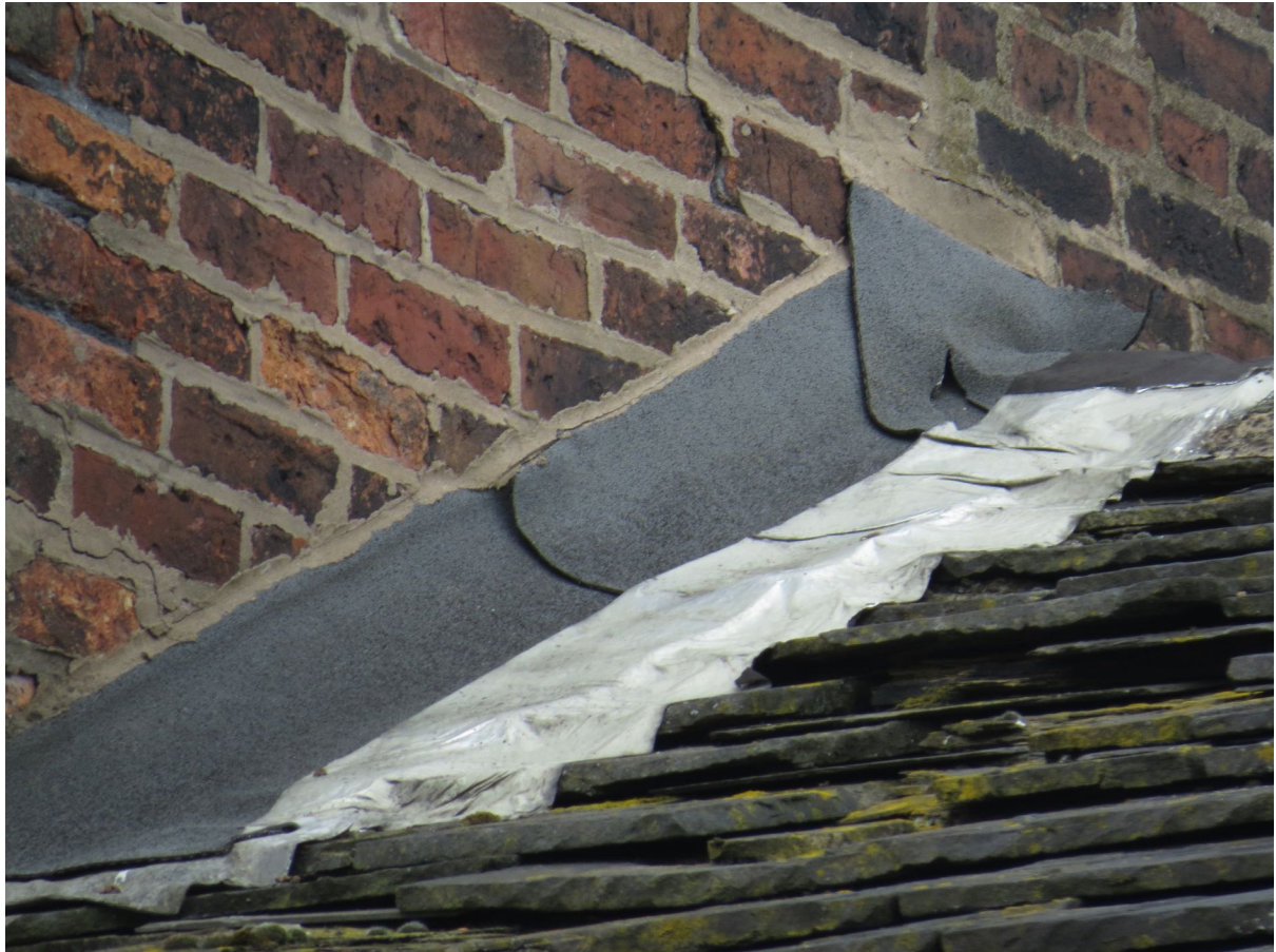
5 – Lead flashing has been replaced with bitumen.
