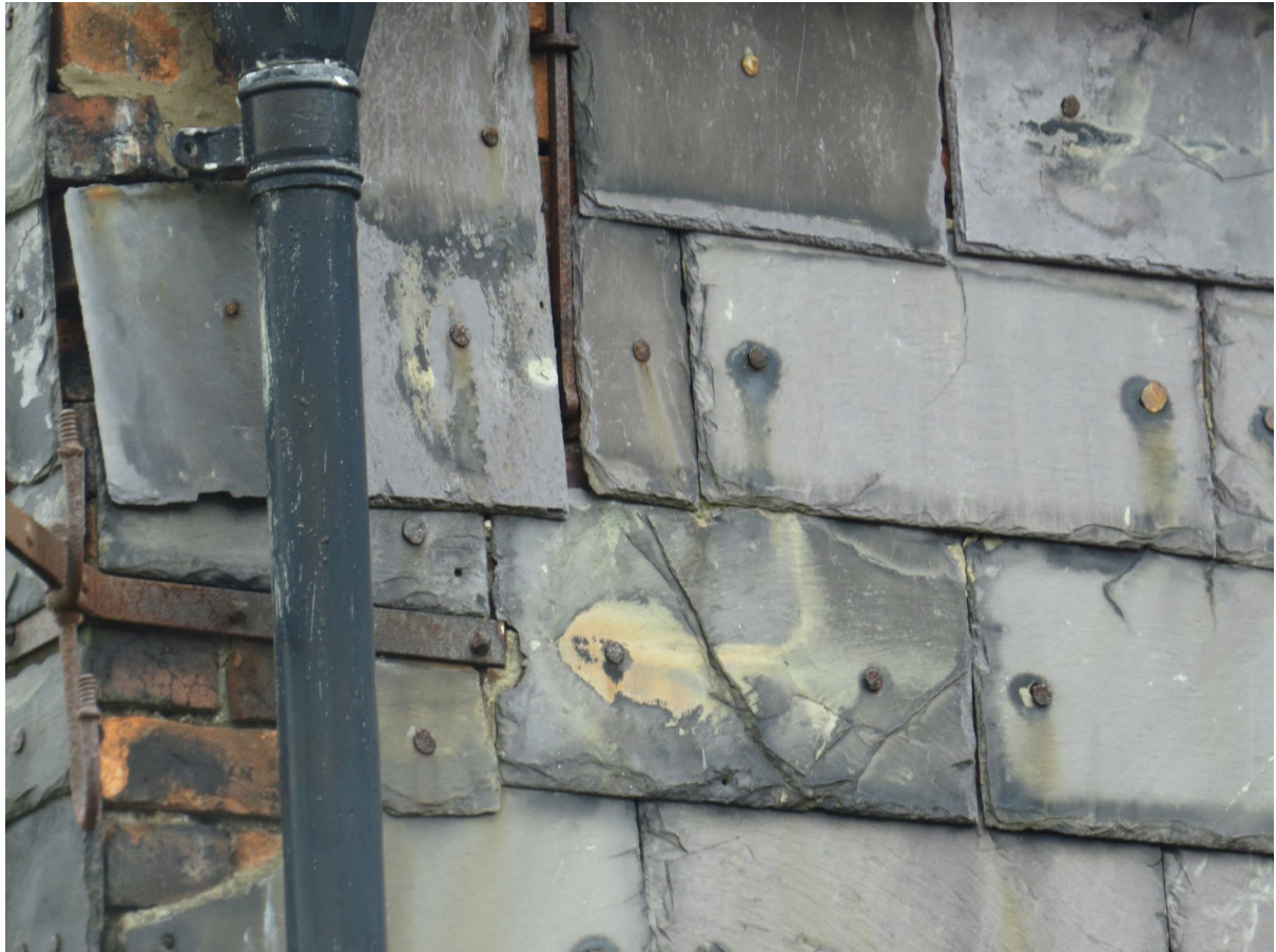
9 – Gaps in hanging tiles were checked from a ladder using an endoscope.
