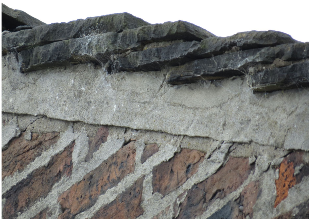
8 – End tiles at the verges are sealed with cement.
