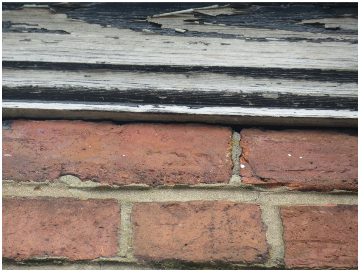
4 – Timber fascia boards at the eaves are fixed tightly against brickwork, but perished.
