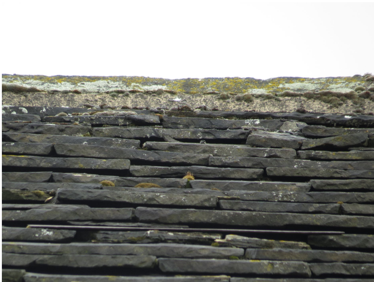
3 – Stone roof and ridge tiles are in good condition.
