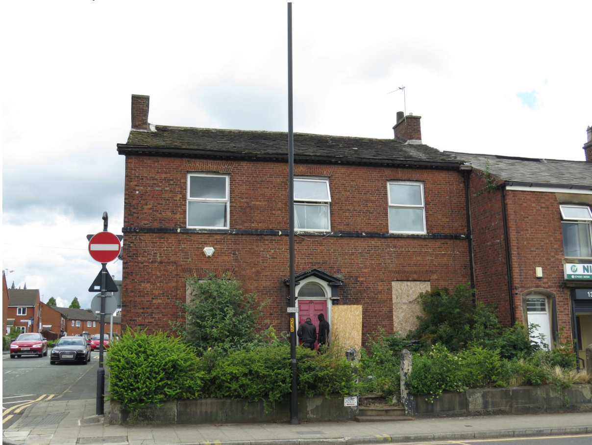
3.1a – The front of the house.
