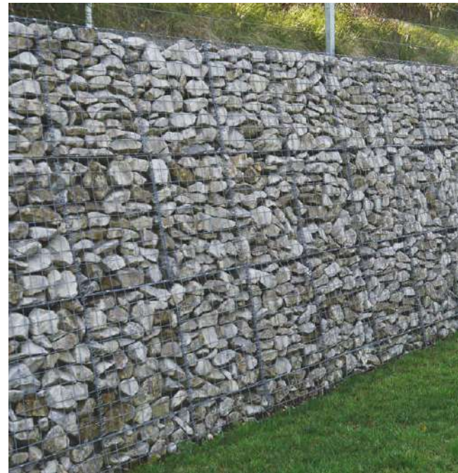
6. Gabion Retaining Wall
