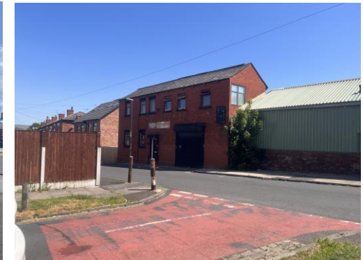
Existing Wham Street Photo (2)
