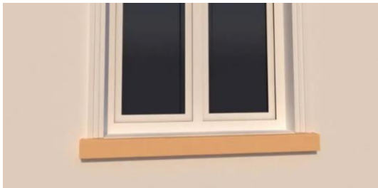
Sandstone window cill.
