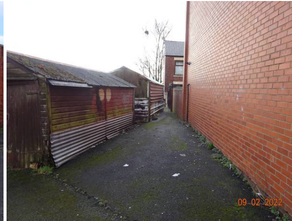
Pic 10 shows the view looking south along the western perimeter of the proposed development site of Block B i.e. the gable wall of no. 3 Grasmere Street.
