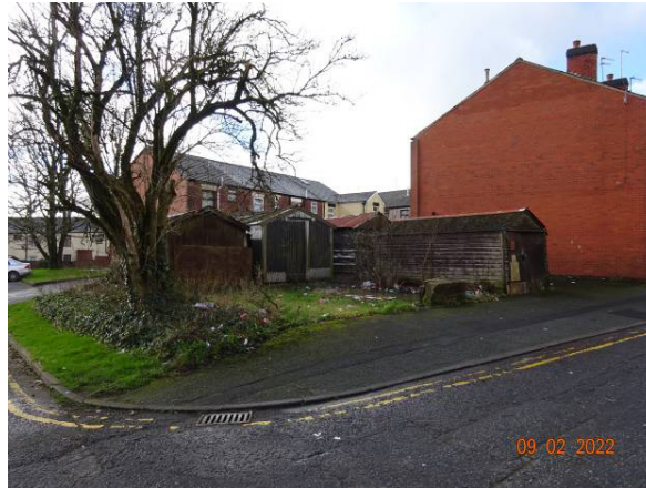
Pic 9 shows the view looking south west across Grasmere Street towards the northern perimeter of the proposed development site of Block B.
