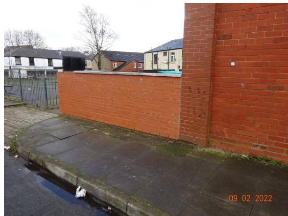
Pic 15 shows an example of one of the existing perimeter treatments to the rear of the established houses seen in Pics 3-5 inc. i.e. a 1.5m high brick wall, the height of which is completely unsuitable for a rear garden /yard as it is easily scaleable.
