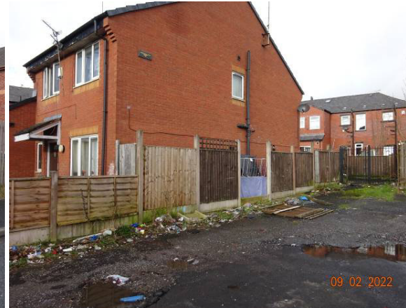
Pic 14 shows the western perimeter of the proposed development site of Block C and its current state of disrepair.
