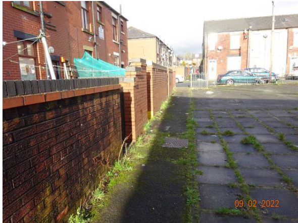
Pic 4 shows the view looking north along the western perimeter of the proposed development site of Block A, with the existing residential properties on Grouse Street on the left of the picture.
