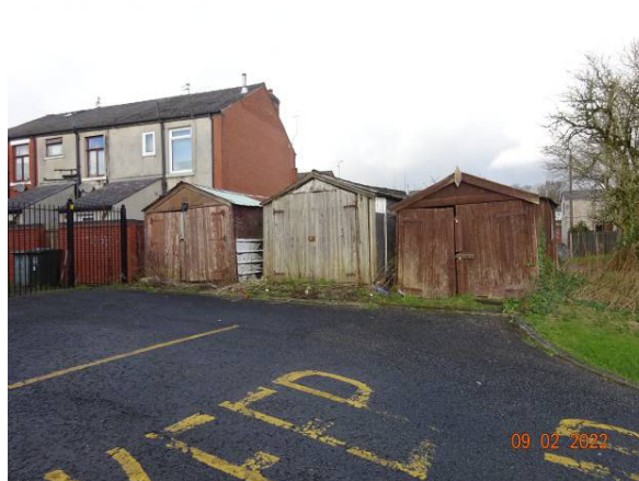
Pic 7 shows the view looking north towards the southern perimeter of the proposed development site of Block B from within the existing car park. The residential properties seen are on Grasmere Street.
