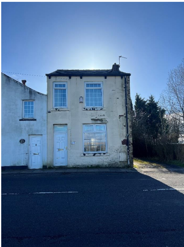
Front elevation of No. 19 Broad Lane
