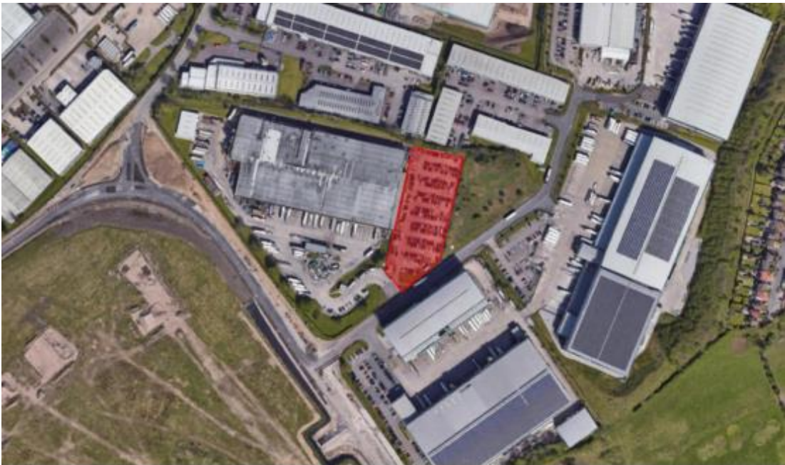
Figure 1.1: Car Park (location highlighted red)
