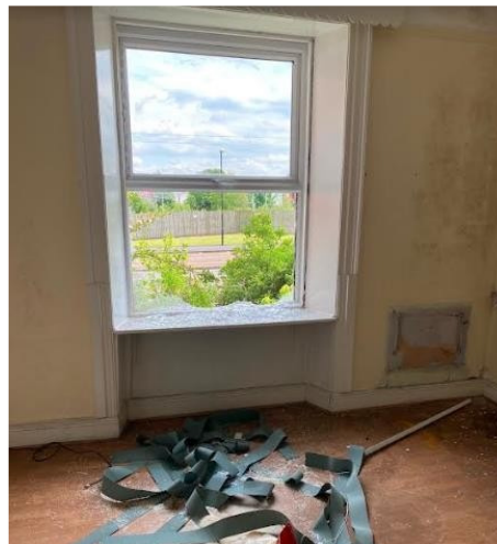
Pl.7: Typical first-floor room and window reveal.
