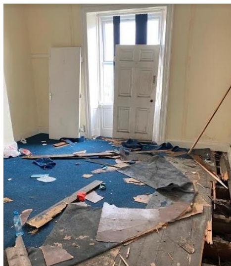
Pl.4: Part of the right-hand front room on the ground floor.
