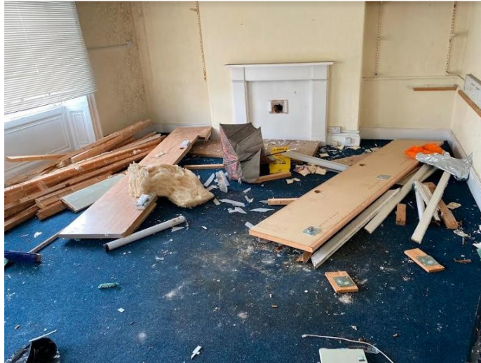
Pl.5: Surviving chimneypiece in the left-hand front room on the ground floor.
