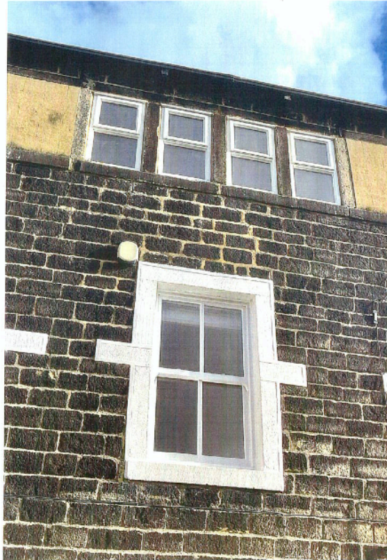
Photograph 3- Existing First Floor and Second Floor Windows
