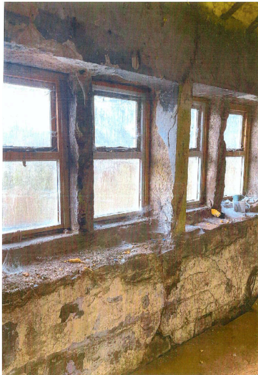
Photograph 4- Existing Second Floor Windows Interior View
