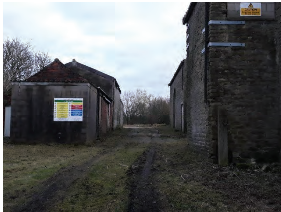
Photo 4—View of derelict Silverhill Farm buildings
