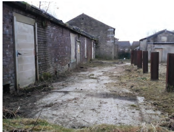
Photo 5—View of derelict Silverhill Farm buildings
