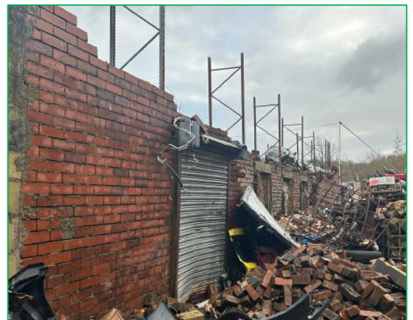
The exposed walls
