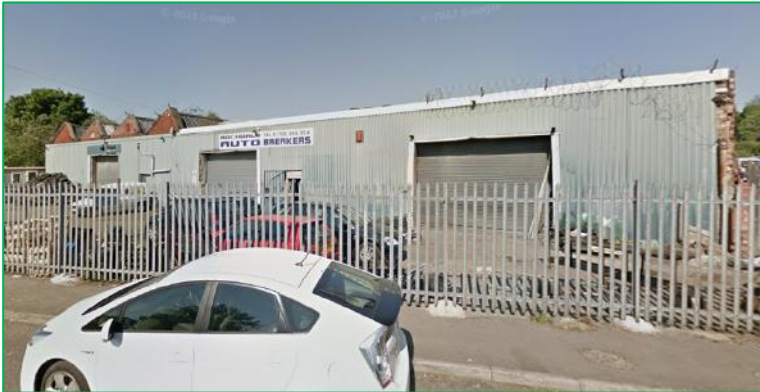
The east elevation of Structure A
