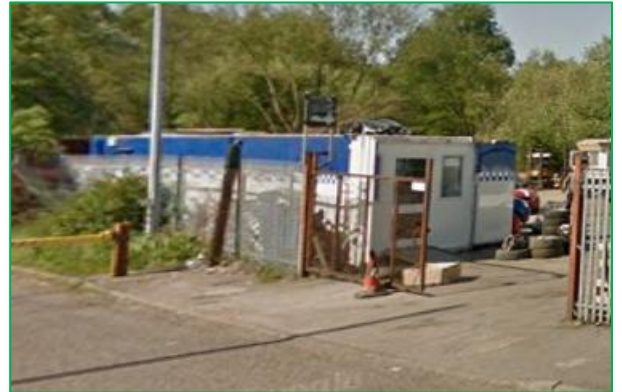
The east and north elevation of Structure B
