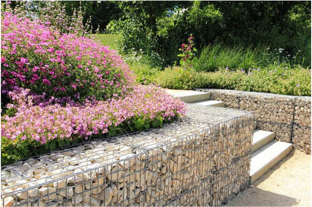
1M high gabion basket retaining walls
