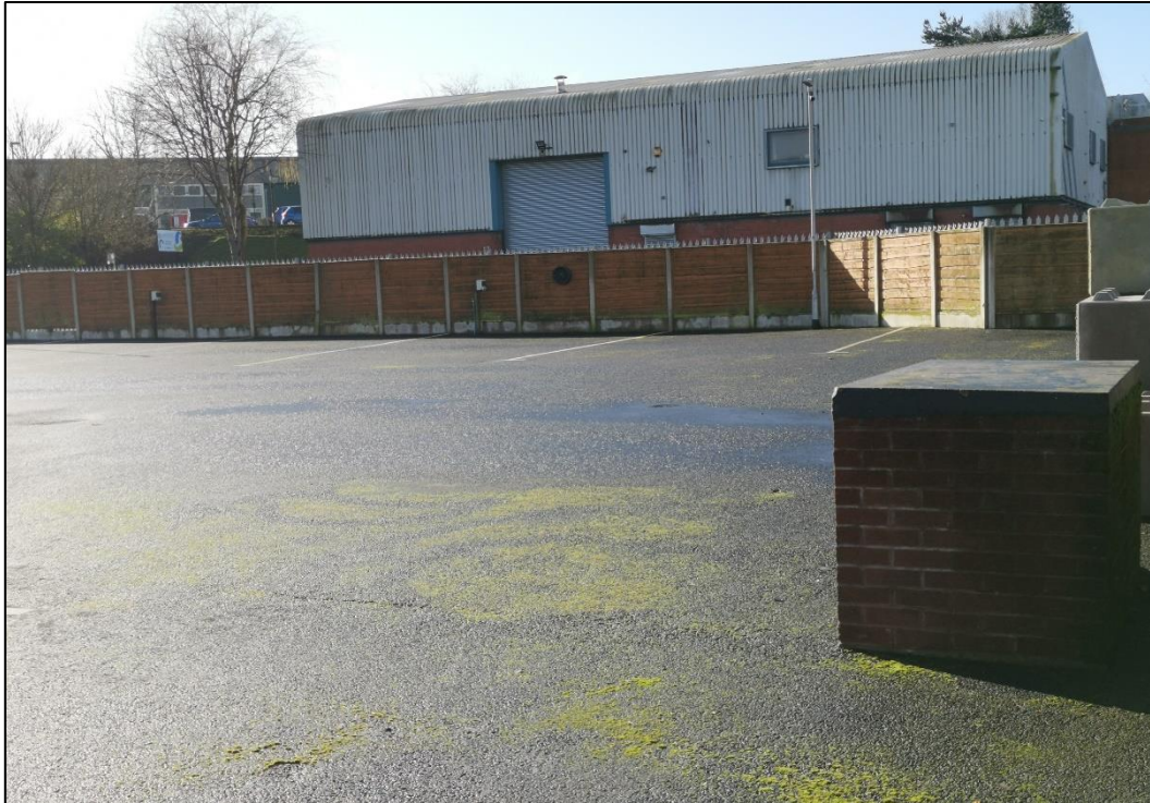
Figure 1 – View to south boundary.
