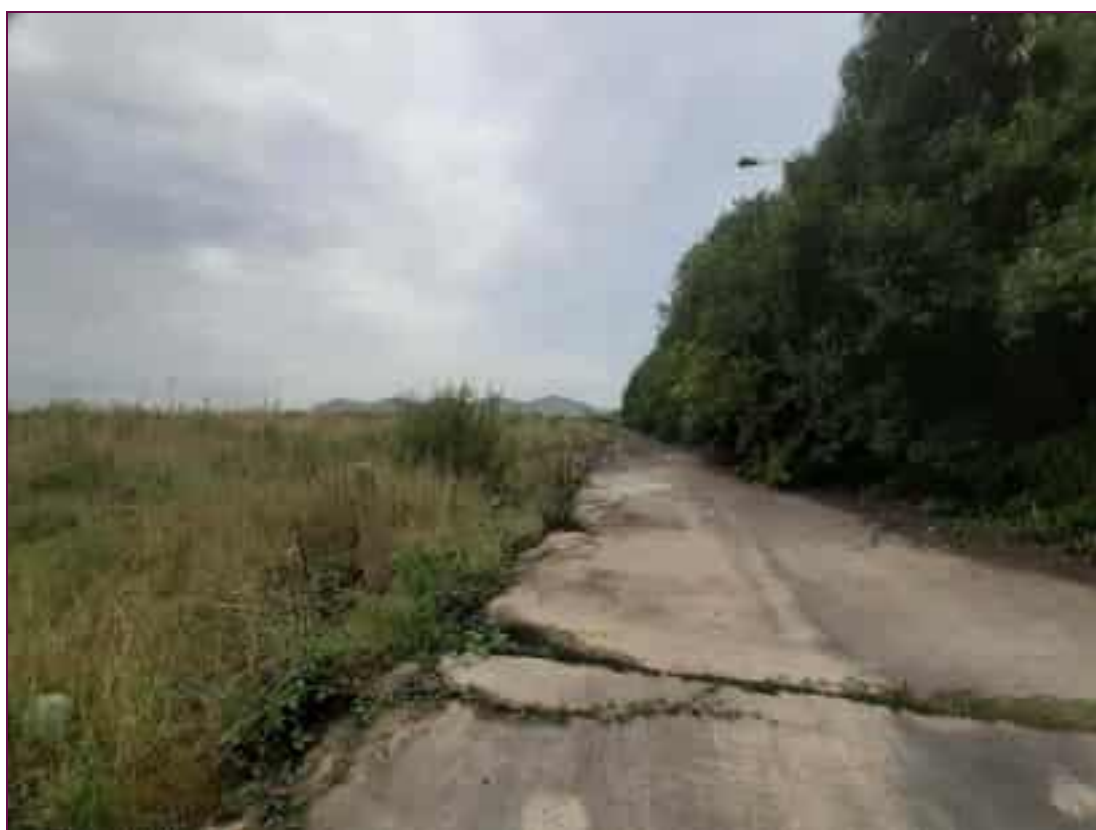
Photograph 8: Concrete Access Road Extending Along Northern Boundary.
