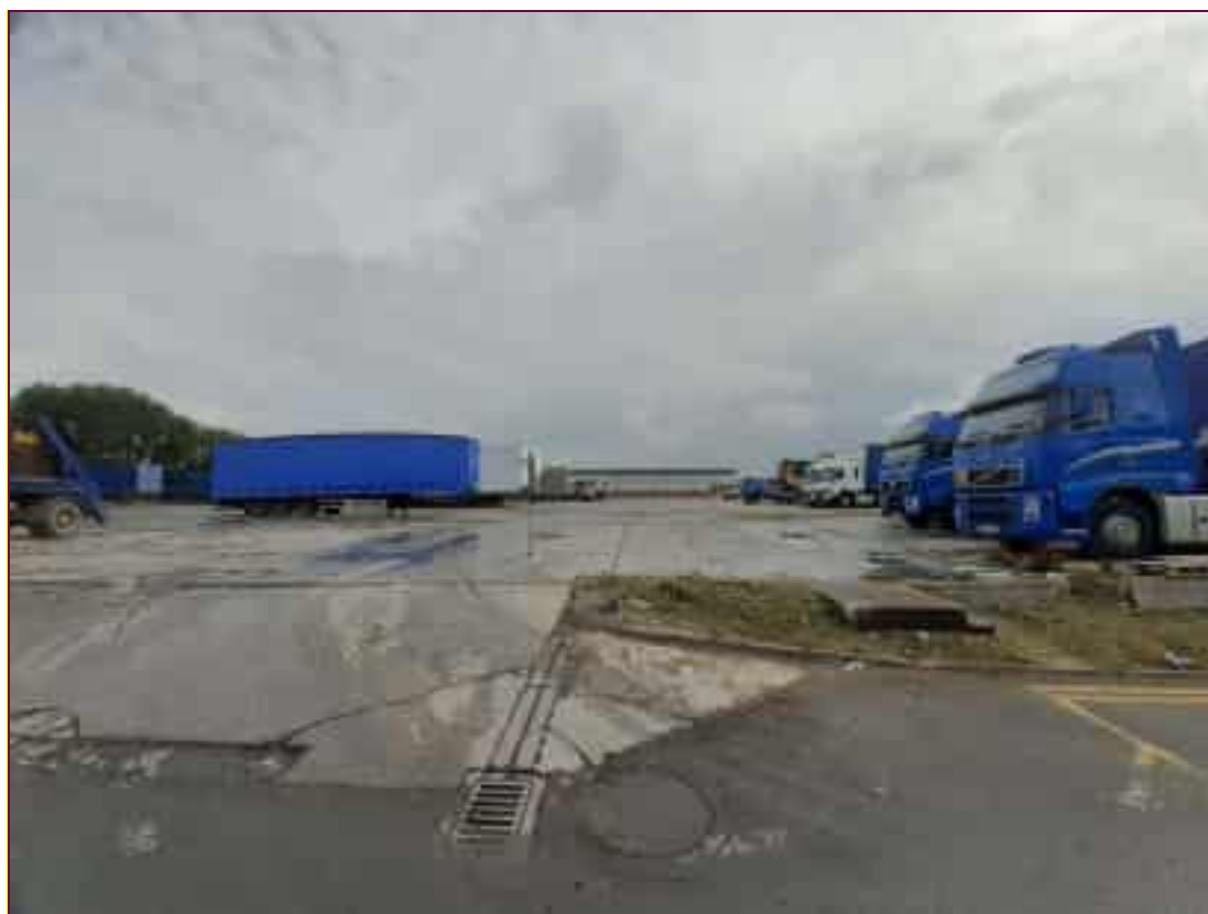
Photograph 1: View from North Looking South-East.
